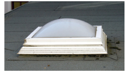
Figure 6. Coupole zénithale scellée
