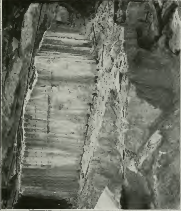
Raising a block of Marble by Shims and Wedges.
