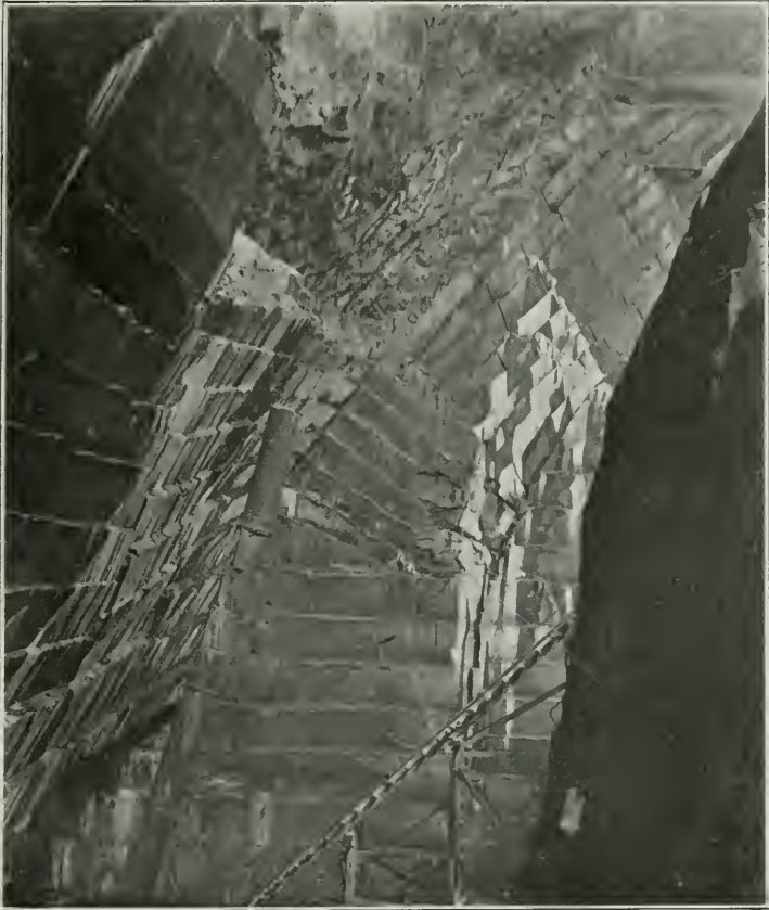
Older part of one of the Quarries at West Rutland, Vt., showing the method of Quarrying on highly inclined beds and the work of the Diamond Boring Channeller.
