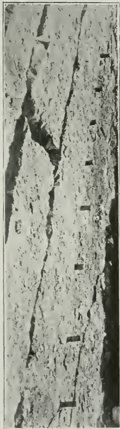
Plug and Feathers in position for splitting rock, Longford Quarries.
