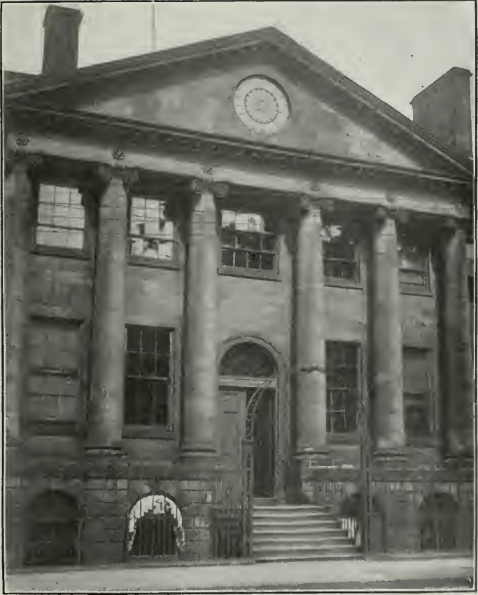
Wallace sandstone. (Batte quarries). Old government buildings, Halifax, N.S
