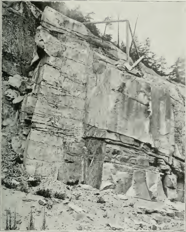
Granite quarry of the Canadian Pacific Railway Co. at Cathmar, B.C.
