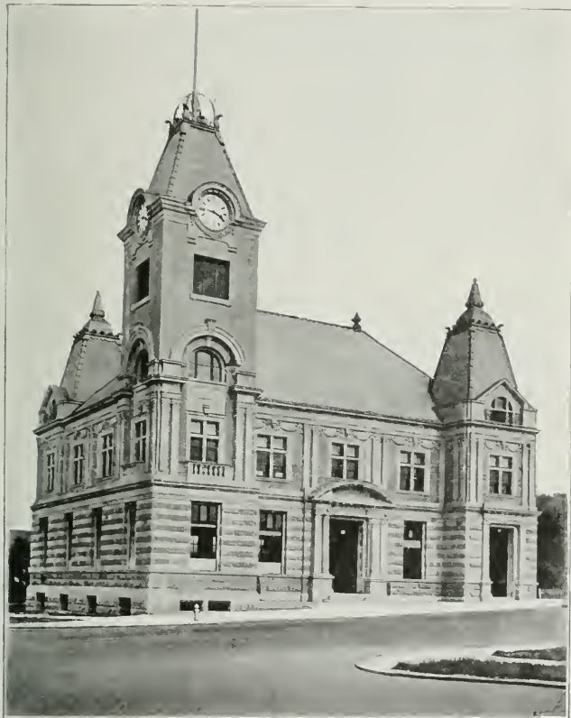
Mayne Island sandstone. Post-office at corner of Main and 15th streets, Vancouver, B.C.
