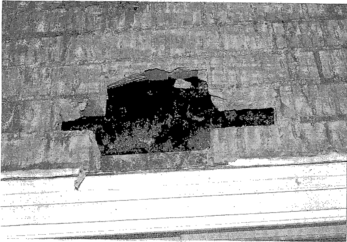
5. Removal of bricks above lintels to inspect flashing
