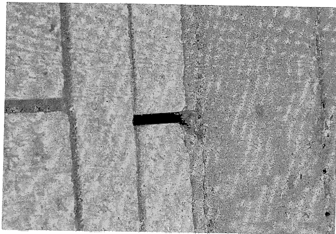
2. Lack of flashing at bottom of exterior wall
