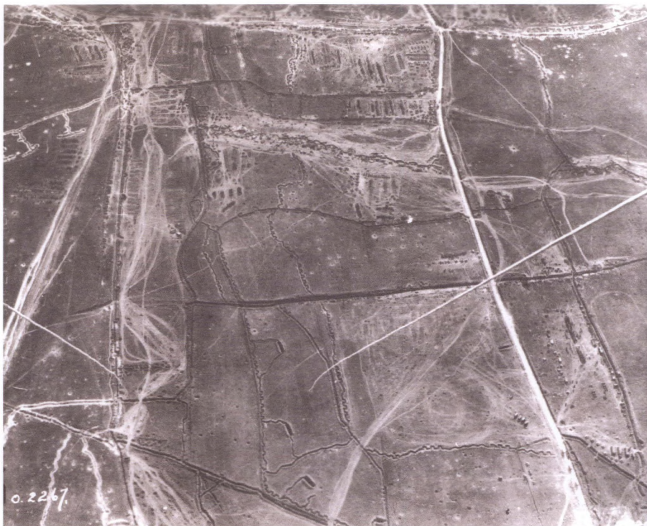
Aerial photographs of the trenches on Vimy Ridge aided military survey units in drafting up-to-date detailed maps of German defences.
