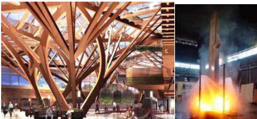
Figure 1 Network of curving glulam beams in the Credit Valley Hospital/Peel Region Cancer Centre in Mississauga and the fire suppression test conducted for the glulam structure using high pressure water mist system (Stanwick, 2003)
