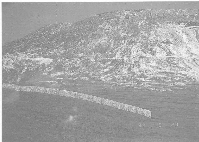
Figure 59 (a) A snow drift near Laramie, Wyoming, photograph by R.D. Tabler. (b) A "Wyoming-style" snow fence along the Dempster Highway in the Richardson Mountains, N.W.T.
