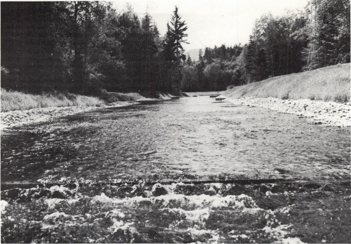
Upstream view of spawning channel adjacent to the river, 1.1 miles from the mouth.
