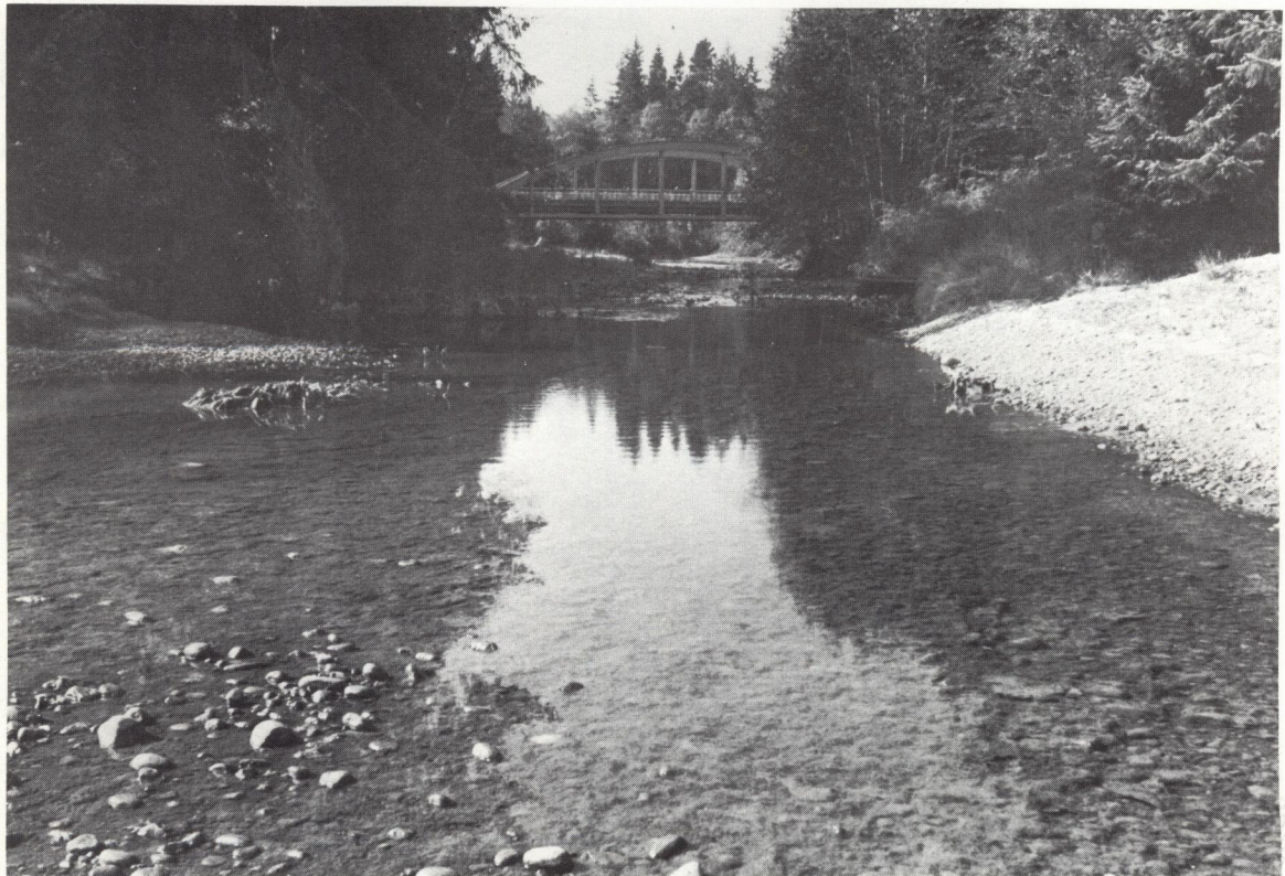
A tidal section of the creek below the highway bridge, 0.4 miles from the mouth.
