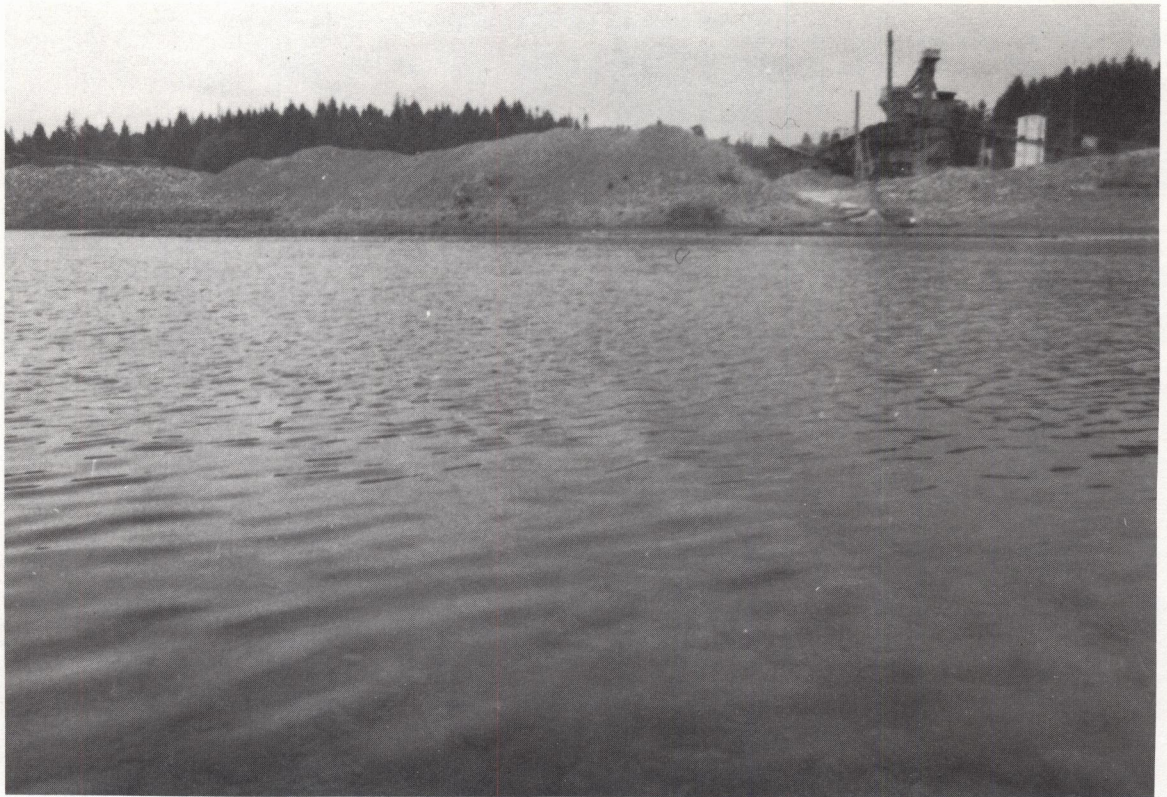
View of LaFarge Cement Co. from across Nanaimo River about one mile from the mouth. LaFarge removes gravel from river for its' operation.
