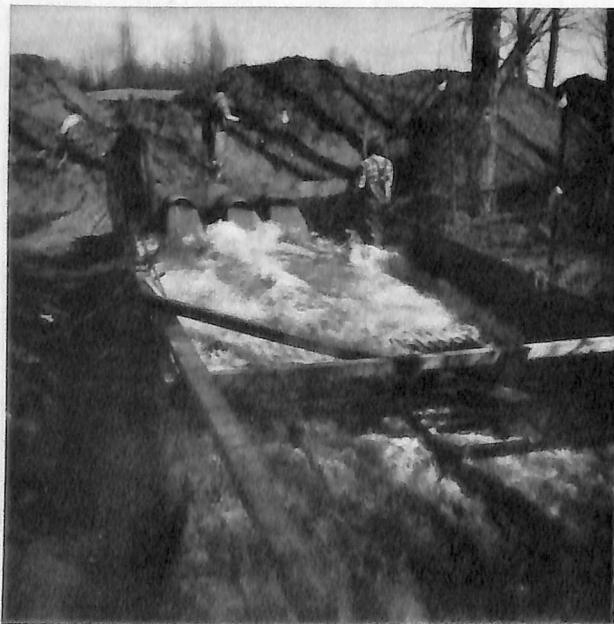
Figure 6. 100% spoil site outflow monitoring, DPW #322 pipeline dredge.
