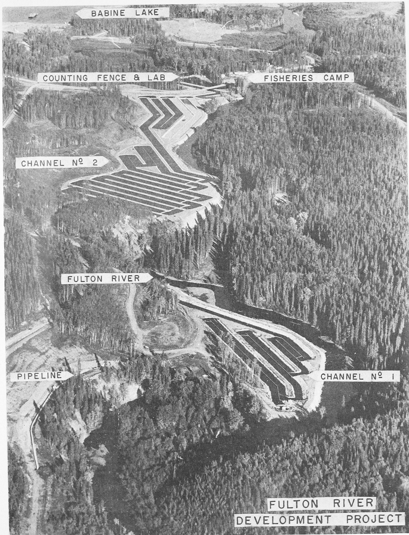
Figure 2: Aerial view of the Fulton River enhancement project.
