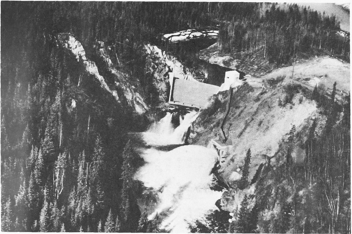
Figure 15: Aerial view of the water control dam located at the outlet of the Fulton Lake reservoir.
