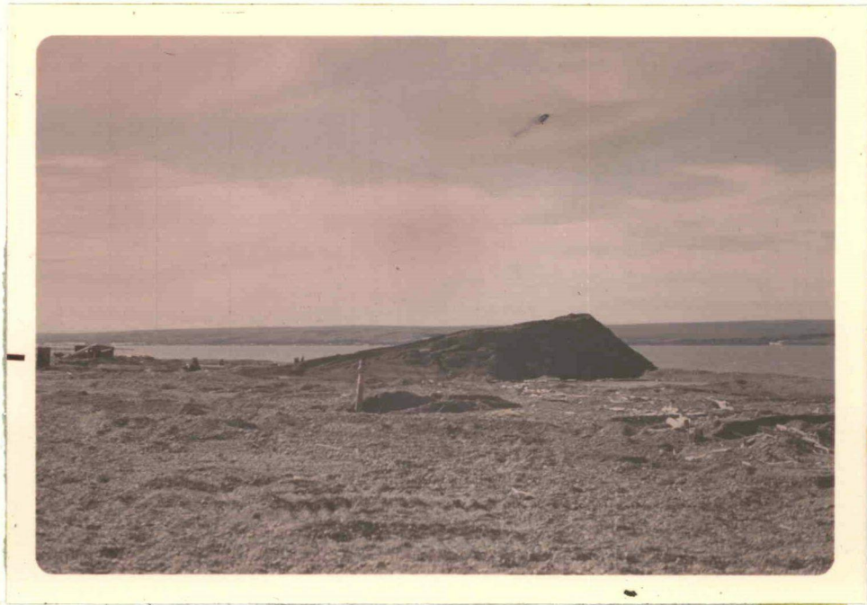
Loading ramp on the shore edge constructed of gravel
