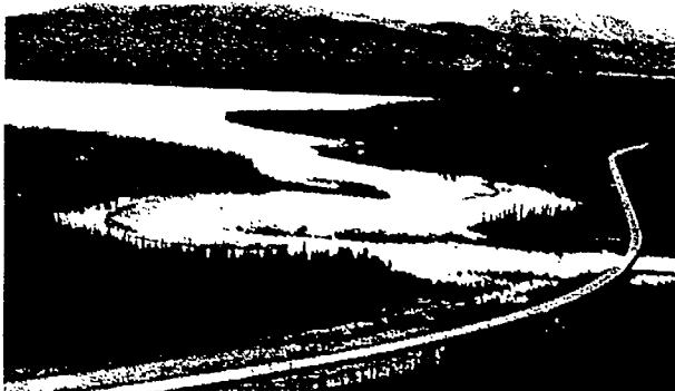
Aerial view downstream of bridge showing flooded area (Photo 9-24A).
