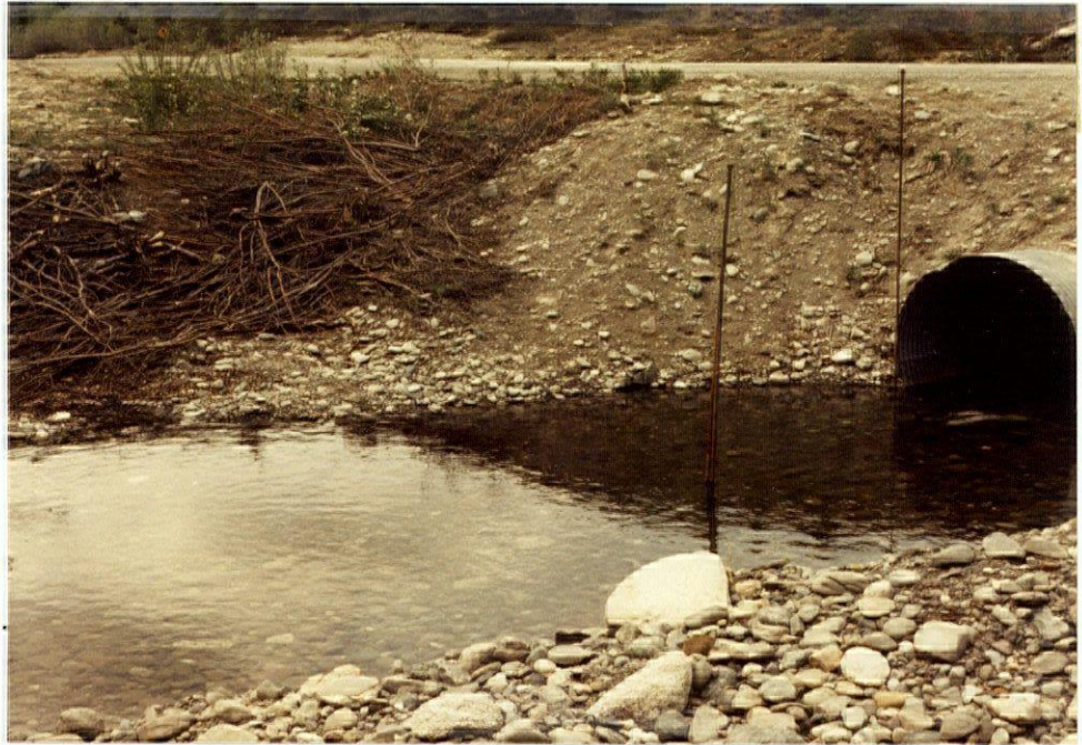
PLATE 81 - If vegetation control is necessary at stream crossings, the least environmental impact is caused by hand clearing methods (km 37, Hwy. 8).
