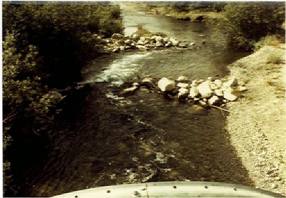
PLATE 69 - Stable rock arrangements in the downstream channel are useful techniques to decrease water velocity and improve fish passage (km 190.6, Hwy. 3).
