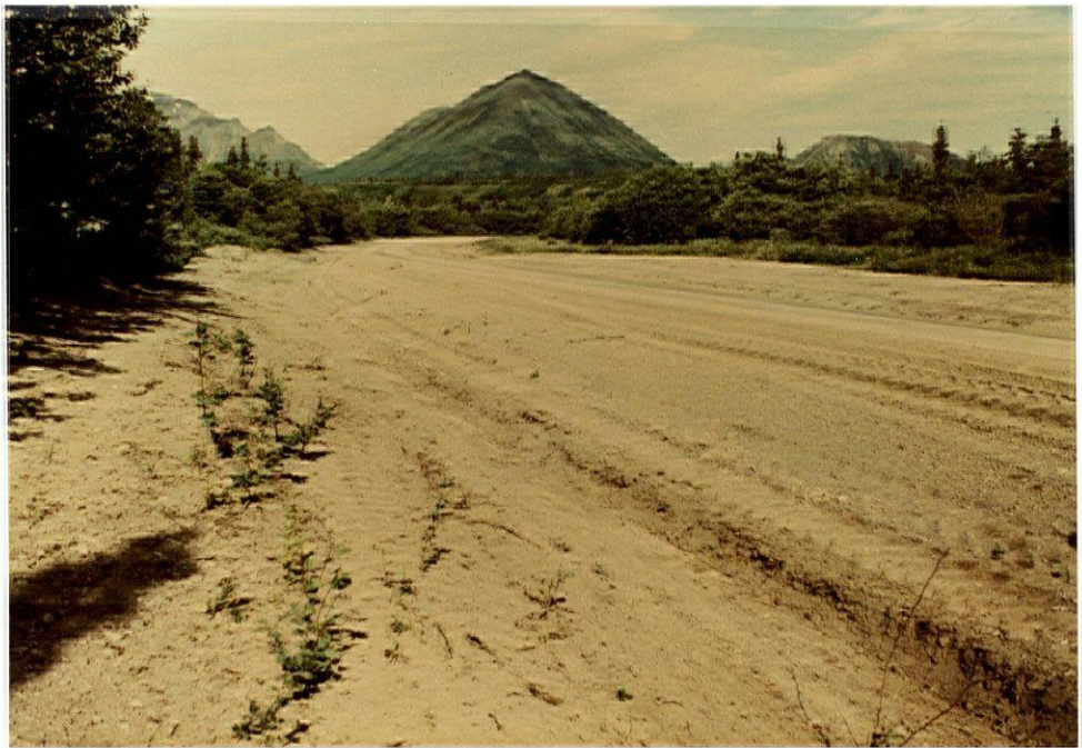
PLATE 82 - Blading the entire right-of-way exposed large areas to surface erosion and conflicts with aesthetic values (km 193, Hwy. 3).
