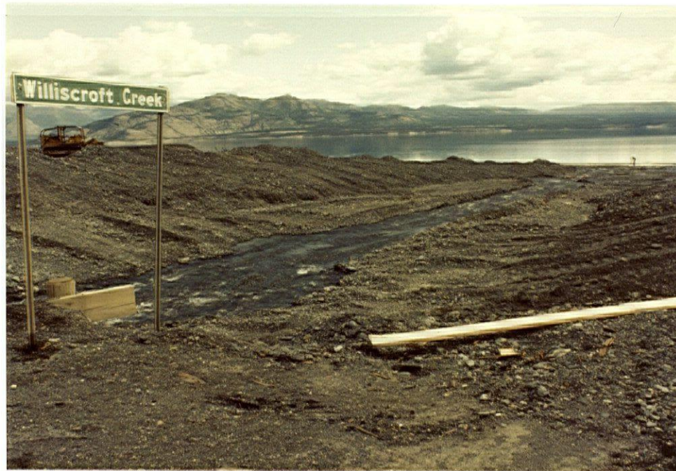
PLATE 74 - The downstream portions of these streams may receive periodic use by fish which reside in the lake. River training programs should be properly planned to avoid possible conflicts with fish utilization (km 1715.8, Hwy. 1).
