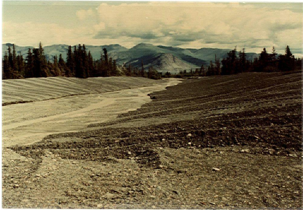
PLATE 73 - Streams with a high bedload movement are dredged for extensive lengths above and below the highway right-of-way to maintain the integrity of the road crossing (km 1724.8, Hwy. 1).
