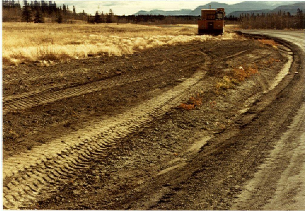
PLATE 83 - Blading in areas which are predominantly grass communities conflicts with good right-of-way management (km 1549.3, Hwy. 1).
