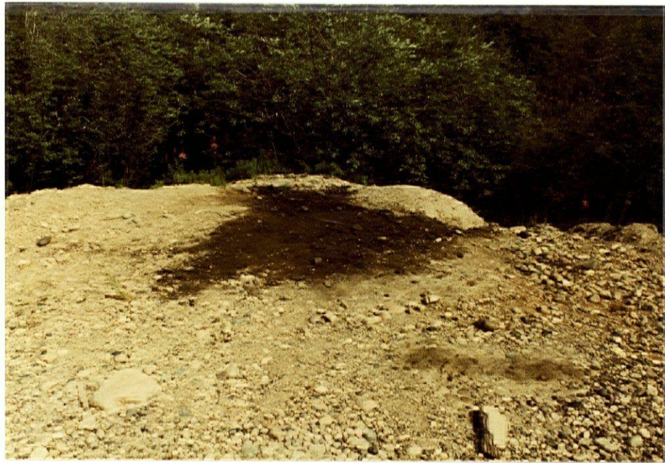
PLATE 77 - Water withdrawal sites should be prepared so that accidental water and oil spills are contained or drain into a vegetated buffer. Oil contaminated soil should be removed to a site where it will not affect water quality (km 637.8, Hwy. 2).
