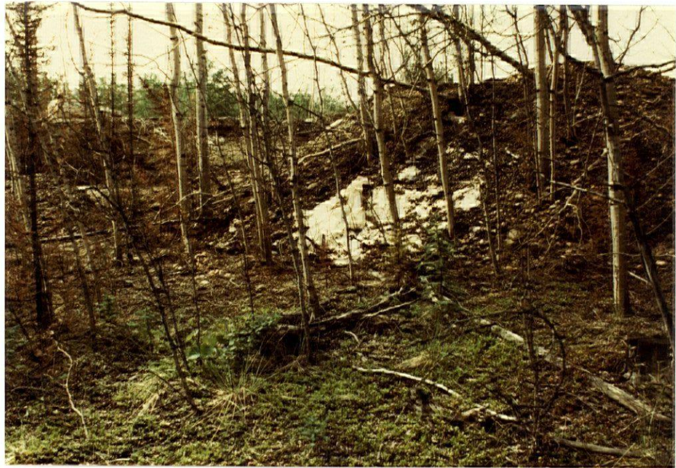
PLATE 75 - Calcium chloride has been inadvertently mixed with overburden material and caused localized killing of the vegetation (km 38.9, Hwy. 11).
