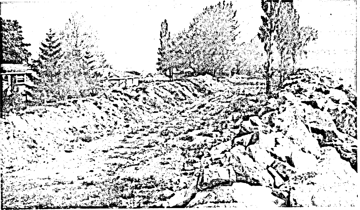
Figure 23 Shore protection, East Beach, Point Pelee. This mile long $800,000 breakwall was built in front of cottages to protect drained agricultural land.
