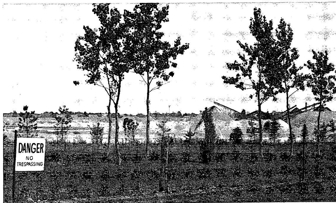
Photo 6. Effective planning is necessary to minimize the impact of pit and quarry operations. Vegetation screens and berms can be useful in visually isolating extraction activities. However, as in this example in Ontario, tree screens planted too late do not always provide as effective a barrier as they might.
