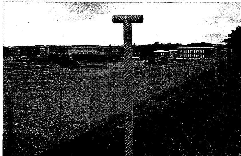
Photo 8. Methane gas proved to be a problem at one Kitchener, Ontario sanitary landfill. These methane gas vents were installed on site to control and disperse the gas. This is particularly important if there are structures nearby. Waste Management Branch, Environment Canada
