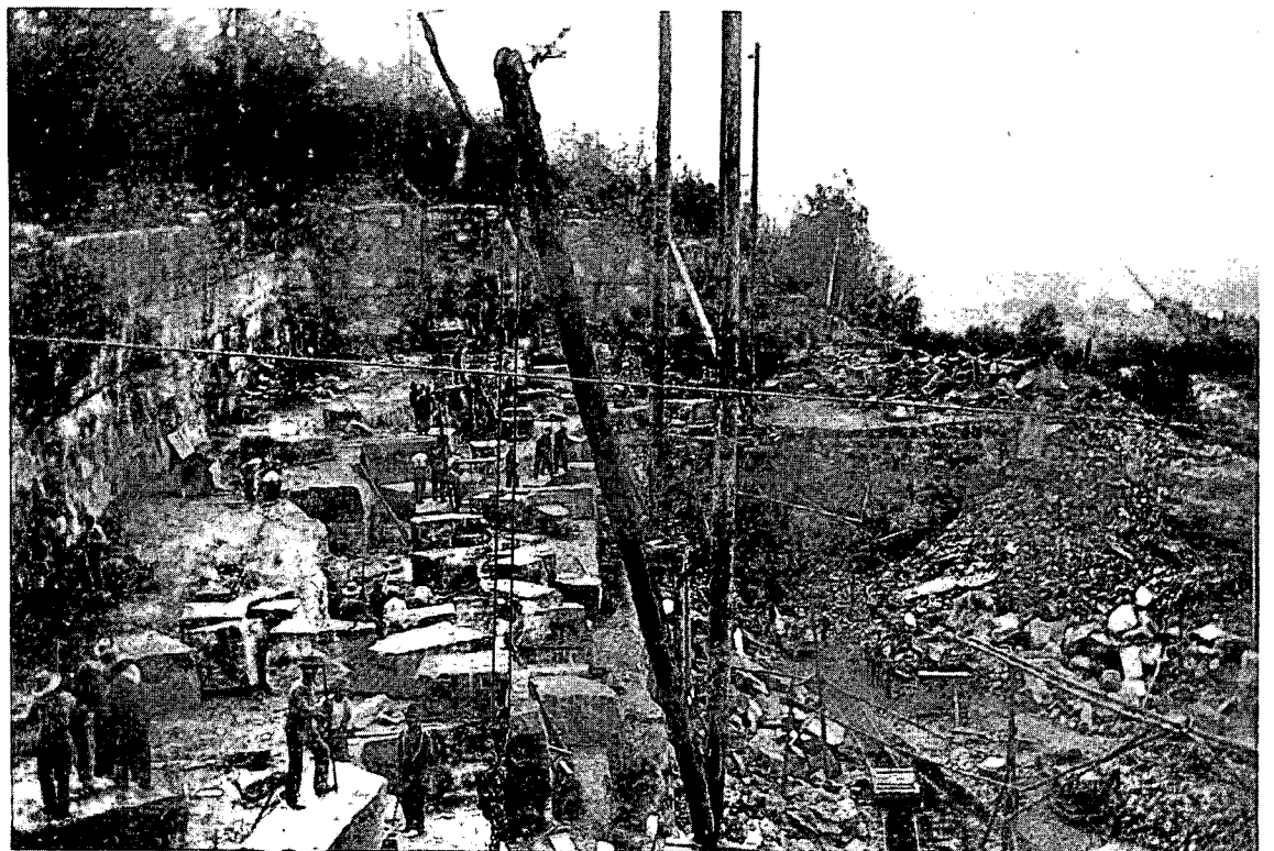
Photo 2. Pits and quarries have a long history in Canada. This 1898 photo of Stewart's Quarry near Rockland, Ontario shows the significant landscape alteration that resulted even without modern extraction equipment.
