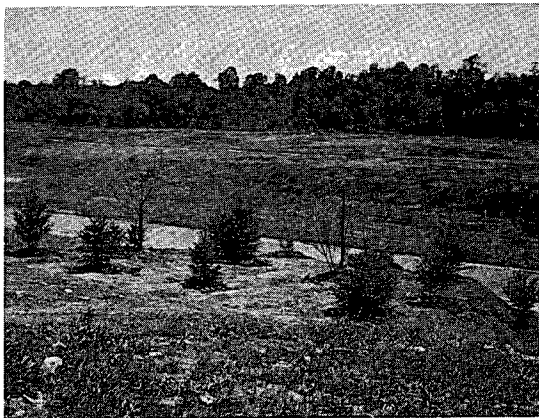
Photo 13. The final soil cover should provide a good basis for re-vegetation and should be contoured to prevent ponding. Grasses and shrubs reduce soil erosion and enhance the visual quality of the rehabilitated site. Waste Management Branch, Environment Canada
