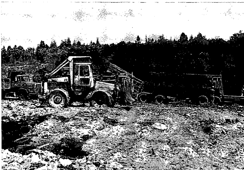
Photo 20. Construction of daily waste cells, June 30, 1981. Fly ash from the Tuft's Cove Thermal Power Station is being unloaded for this, a special permit from the Nova Scotia Department of the Environment was required. E. Kienholz, Lands Directorate, Atlantic Region
