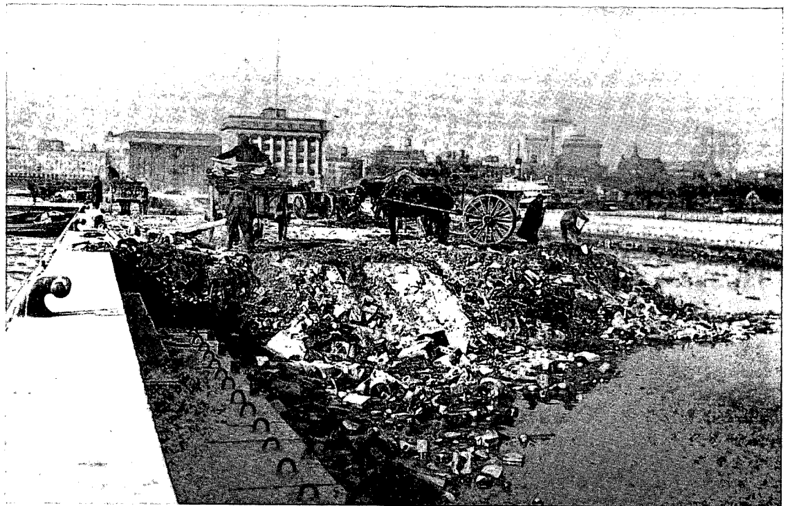
Photo 1. This garbage dump at the Toronto waterfront in 1922 illustrates the waste disposal technique and philosophy that existed at that time.
