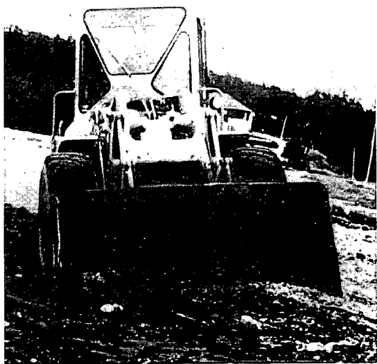
Photo 10. Wheeled front-end loader removing a wide (5 m) thick (10–20 cm) layer of oil deposited at the high-water level on a pebble-cobble beach in southern Chedabucto Bay, April, 1970. E.H. Owens
