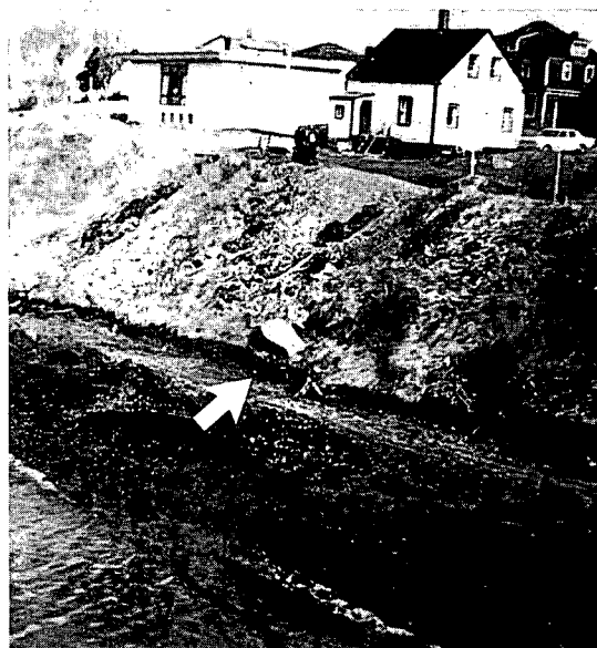
Photo 9. Cliff of unconsolidated material at Arichat, Nova Scotia. Initial removal of oil and sediments from the intertidal zone by a bulldozer removed the protective beach and cut a notch (arrow) at the base of the cliff. This could easily have resulted in erosion of the cliff by wave action and consequent damage to property if remedial action had not been taken.
