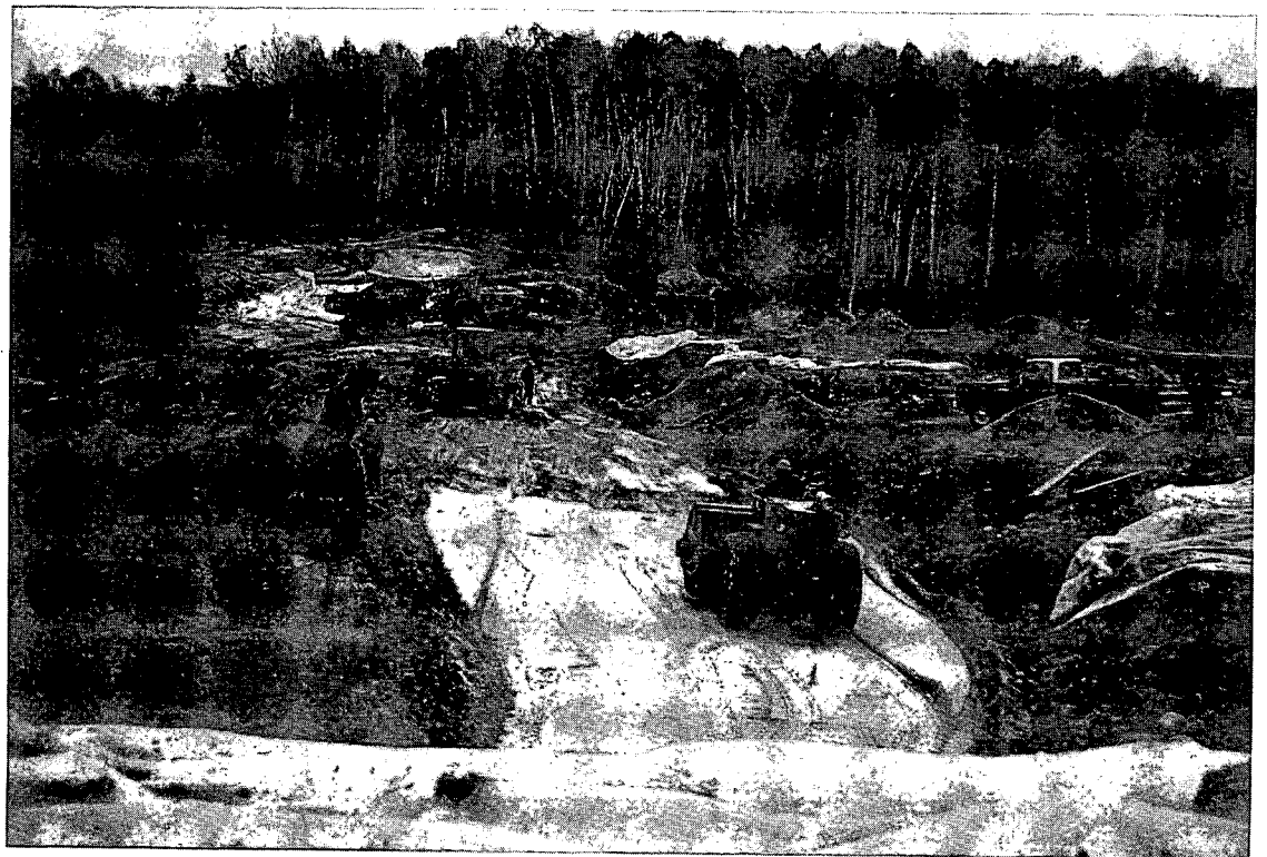
Photo 6. Work on tailings. I.G. Redmond
