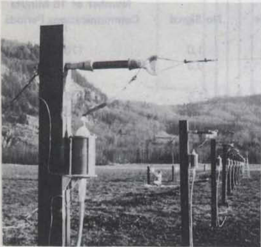
Matching Transformers at Feed End
