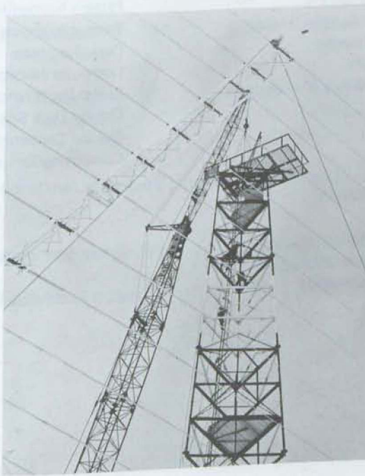
The assembly of 6 — 40 MHz log-periodic antenna by CRC Plant Engineering Services.
