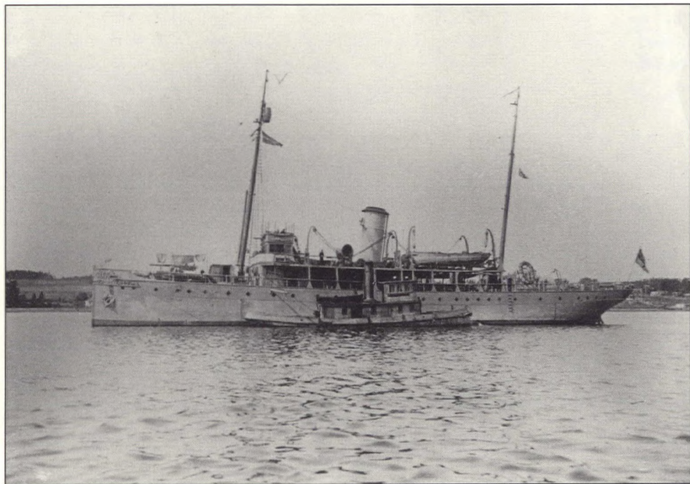
Although HMCS Acadia , seen here in September 1918, was not formally commissioned until 1917, the hydrographic vessel had performed naval duties since 1914. She carried a 4-inch gun forward but her usefulness as a patrol vessel was hampered by her eight-knot top speed. (LAC e007140896)
