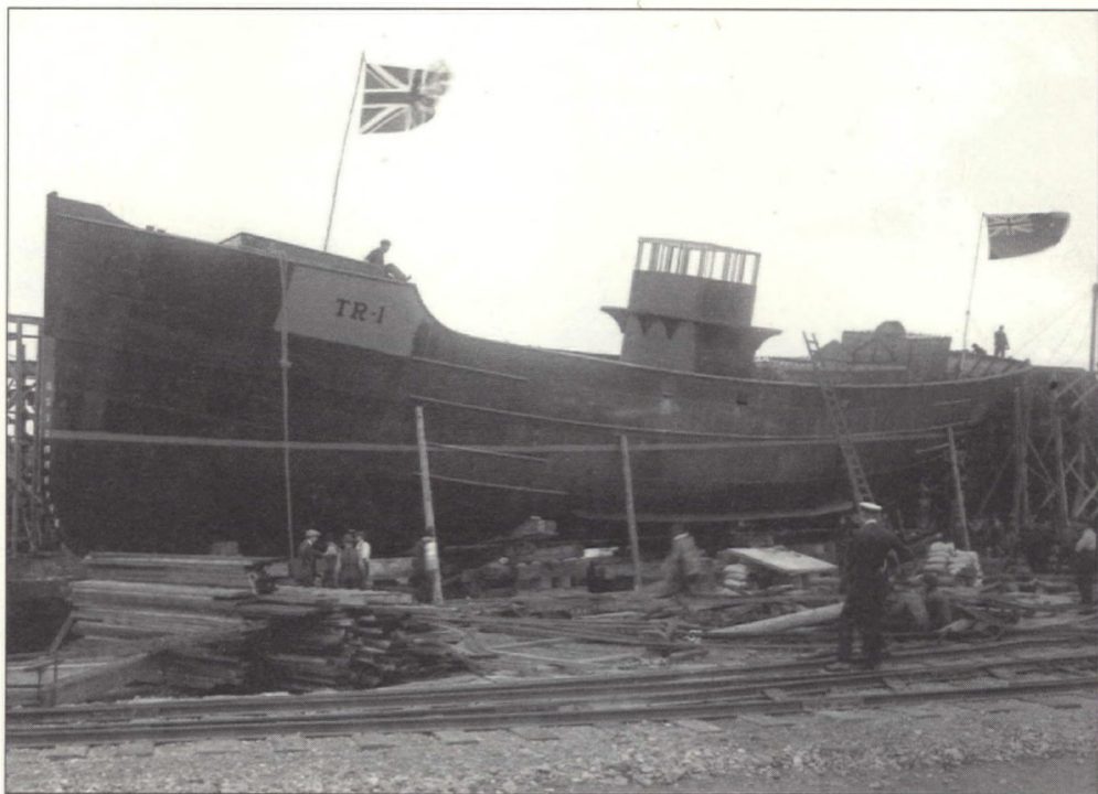
The first of the thirty-six Imperial trawlers ordered by the Admiralty, TR 1 , under construction at Port Arthur, Ontario, in 1917. (LAC B-002994)
