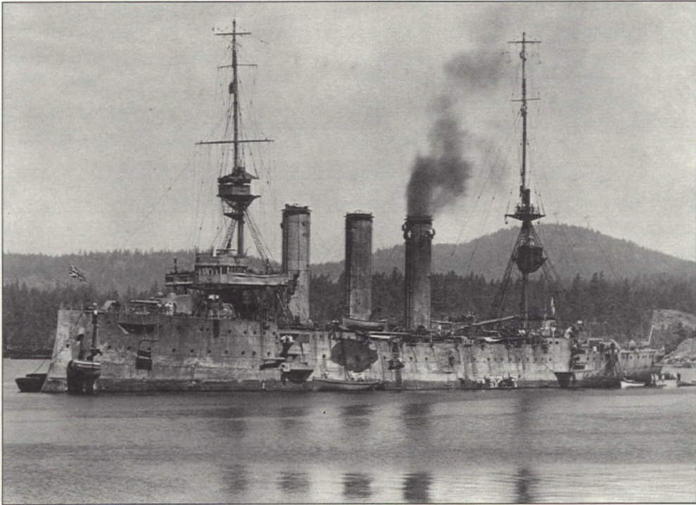
The cruiser HMS Cornwall at Esquimalt repairing some of the eighteen hits she received at the Battle of the Falkland Islands on 8 December 1914 where she sank the German cruiser Leipzig . Cornwall was a sister ship to HMS Monmouth , sunk at the Battle of Coronel. (DND E-38800)
