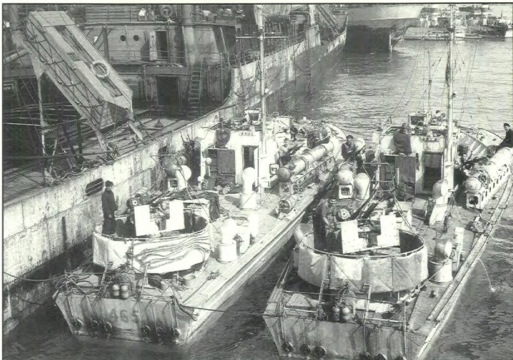
Short motor torpedo boats of the 29th MTB Flotilla. With a crew of three officers and fourteen ratings, the seventy-two-foot-long boats had a top speed of more than thirty knots. (DND JT-307)
