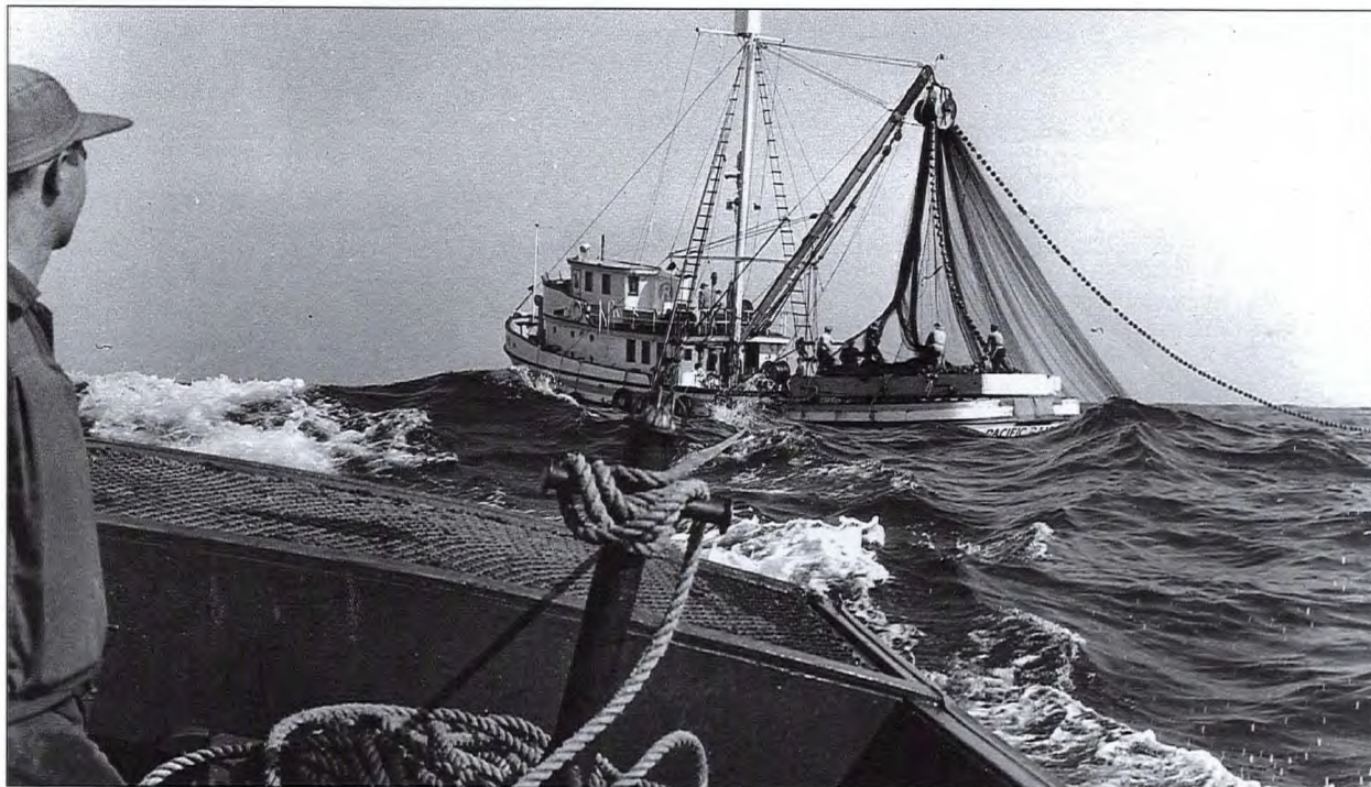
As on the Atlantic, bigger, better boats were the trend. In the seine fleet, "table" seiners, with the net stowed on a turntable for easier running, dominated at first. Here, the Western Ranger , seining for sockeye in 1958, has completed a set. The power skiff tows the vessel from the side, to keep her from drifting into the floating seine while taking it in. (Library and Archives Canada, PA-146255)
