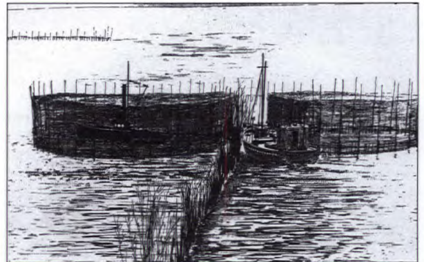
A pumper inside the weir and a carrier entering. (Walter Scott drawing)
