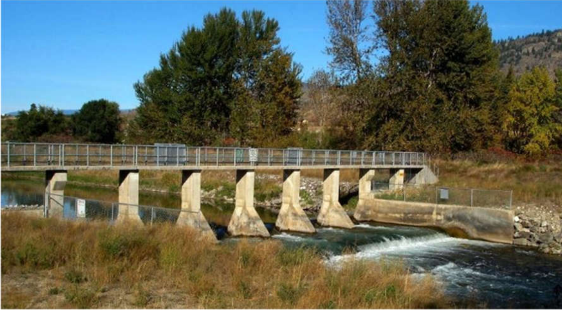
Figure 2. Example of a Vertical Drop Structure on the Okanagan River, B.C.
