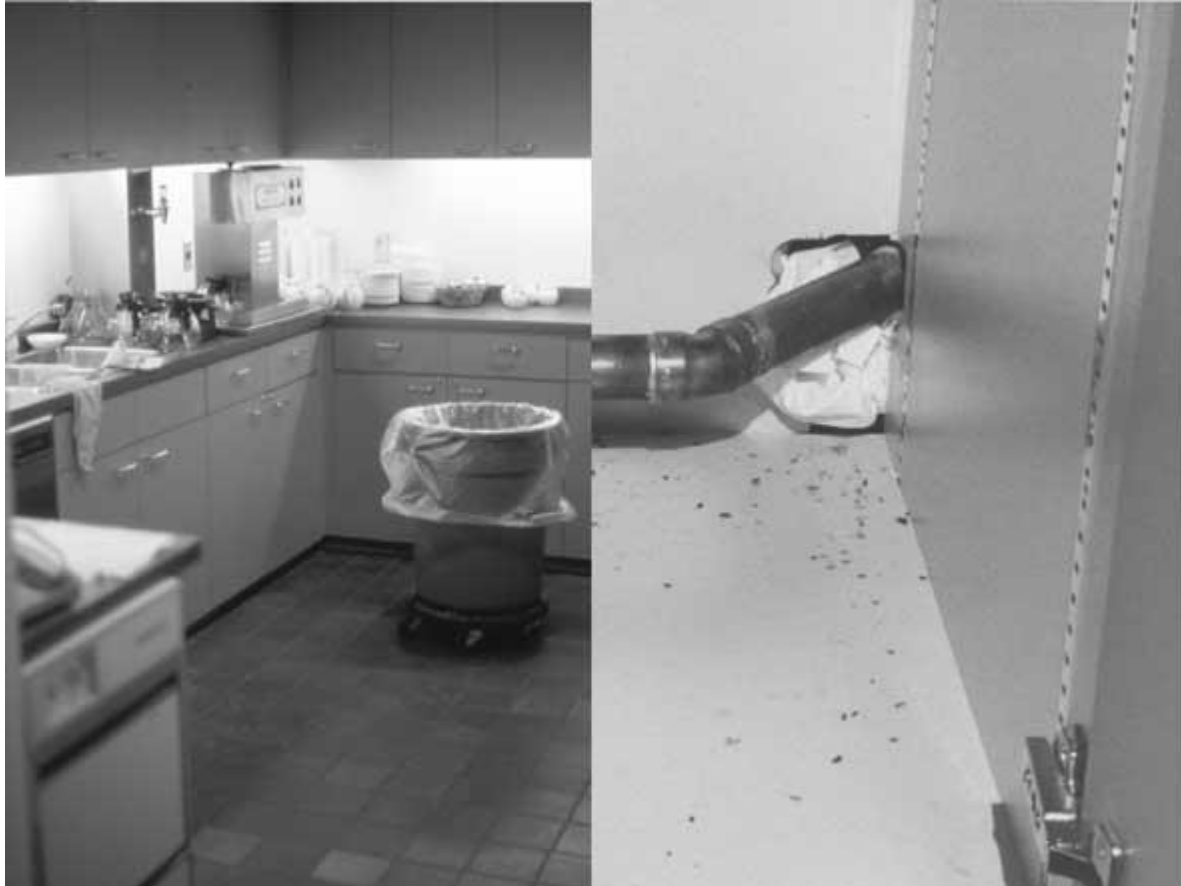
Figure 11. Kitchens are attractive to rodents, which can enter through a badly fitting pipe chase or by crawling under doors. Most rodent problems are associated with human food in buildings. On the right, mouse feces can be seen in the cupboard. The access hole has been ineffectively plugged with crumpled paper.
