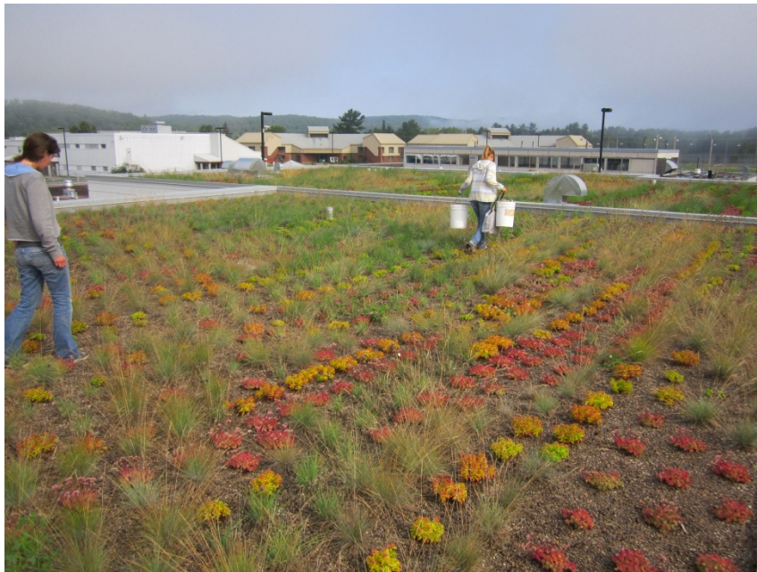
Green roof on infirmary, La Macaza, Quebec Region
