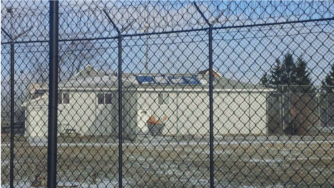
Solar hot water project on a Private Family Visit building, Bath Institution, Ontario Region.
