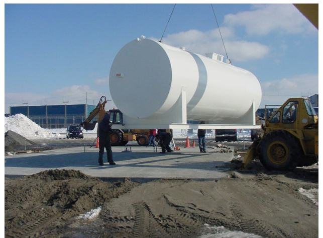
Petroleum Storage Tank Replacement Drummond Institution, Quebec Region
