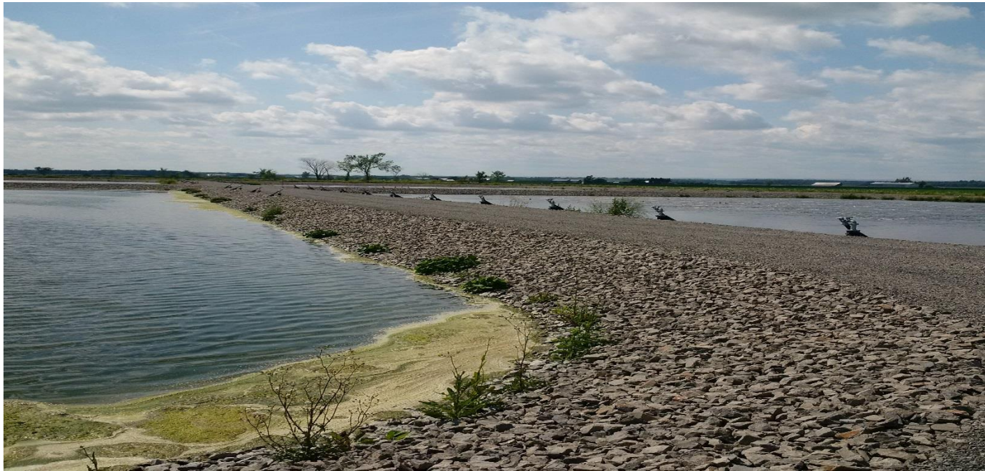
Tree planting at the wastewater lagoon at SADP Institution, Sainte-Anne-des-Plaines, QC.
