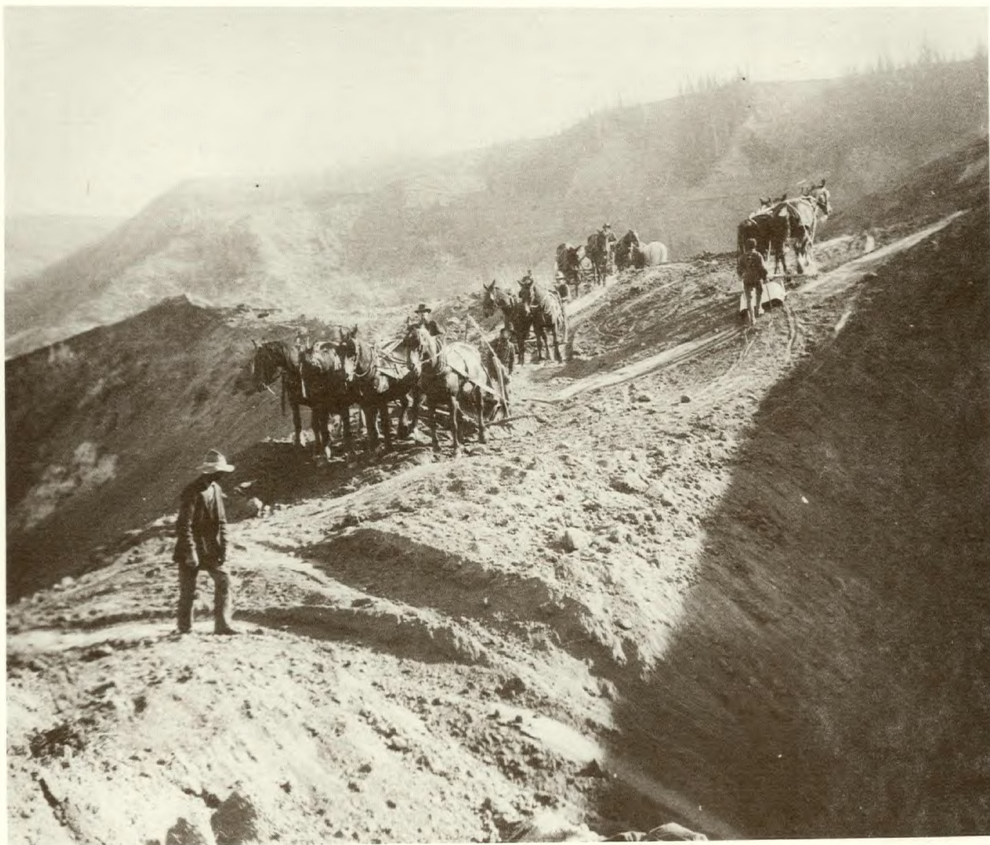
121. Railway grading, Alberta. According to the Canadian Annual Review for 1907, 5,800 miles of railroad were under contract between the Great Lakes and the Rocky Mountains. Included were 1,500 miles of the Canadian Northern, 1,400 miles of the Canadian Pacific, 1,000 miles of the Great Northern and 1,900 miles of the Grand Trunk Pacific. By September 1907, approximately 3,000 miles were actually under construction.
