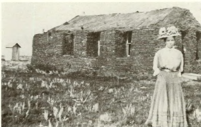
77. Sod house, Saskatchewan.
