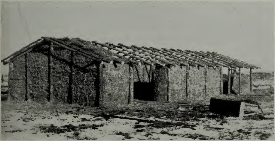
Straw shed partially completed.
