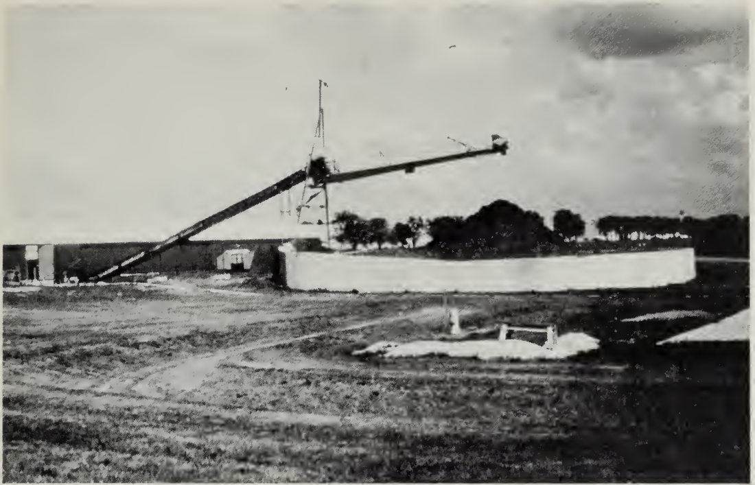
Fig. 8. Proper manure-storage facilities such as these help prevent dilution of the manure. Surface runoff and roof runoff are rerouted away from the storage area. In areas with high precipitation a roof might be necessary to keep excess water out.
