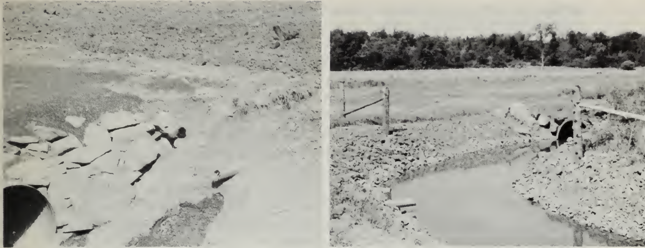
Fig. 6. The tile outlet, culvert headwall, and unvegetated ditchbank pictured on the left all contribute to increased soil erosion.
