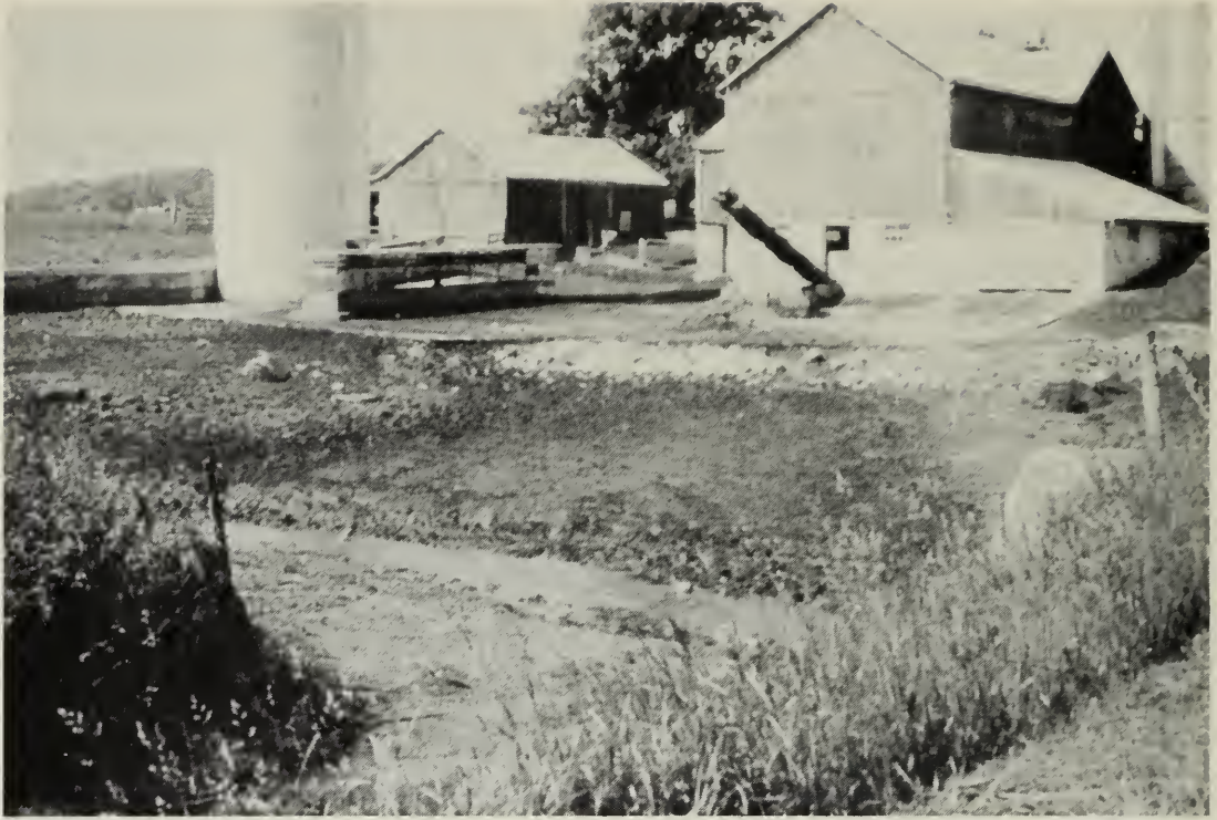
Fig. 7. Manure storage areas and livestock yards that are not adequately separated from ditches and streams, either by distance or structural means, reduce the quality of the local water.
