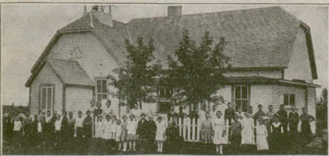
There is not a Settled Township without a School
