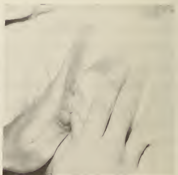
Figure 15. Pressing the adhesive-coated surface of the bag into place.
