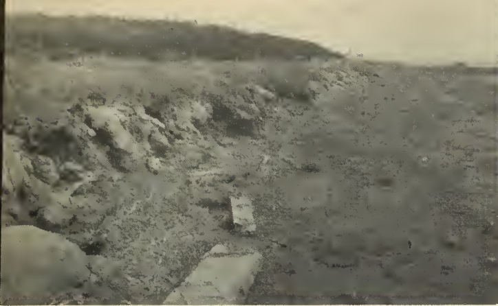
Left: Severe erosion of exposed dike face, Beaumont, N.B. Right: Tall wheat grass growing on a dike at Nappan, N.S. Note grass well below high tide level indicated by stake and debris.
