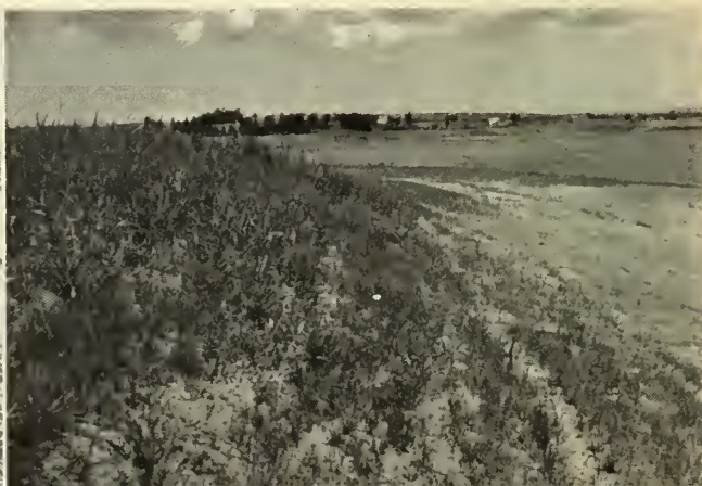
Left: Spraying bituminous emulsion on newly seeded outer slope of dike, Westcock, N.B. Right: Side of dike showing catch of grass.
