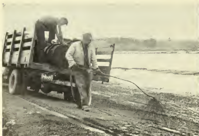
Left: Spraying bituminous emulsion on newly seeded outer slope of dike, Westcock, N.B. Right: Side of dike showing catch of grass.
