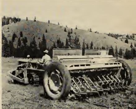
Seeding depleted grasslands with the Oregon Rangeland Drill. Each 20-inch disc is on a pivoted arm and has sufficient weight to carve a furrow even in uncultivated rangeland.
