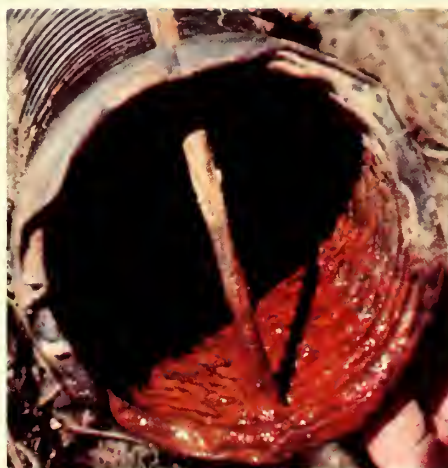
Figure 1. Close-up view of a tile outlet showing red, slimy effluent.
