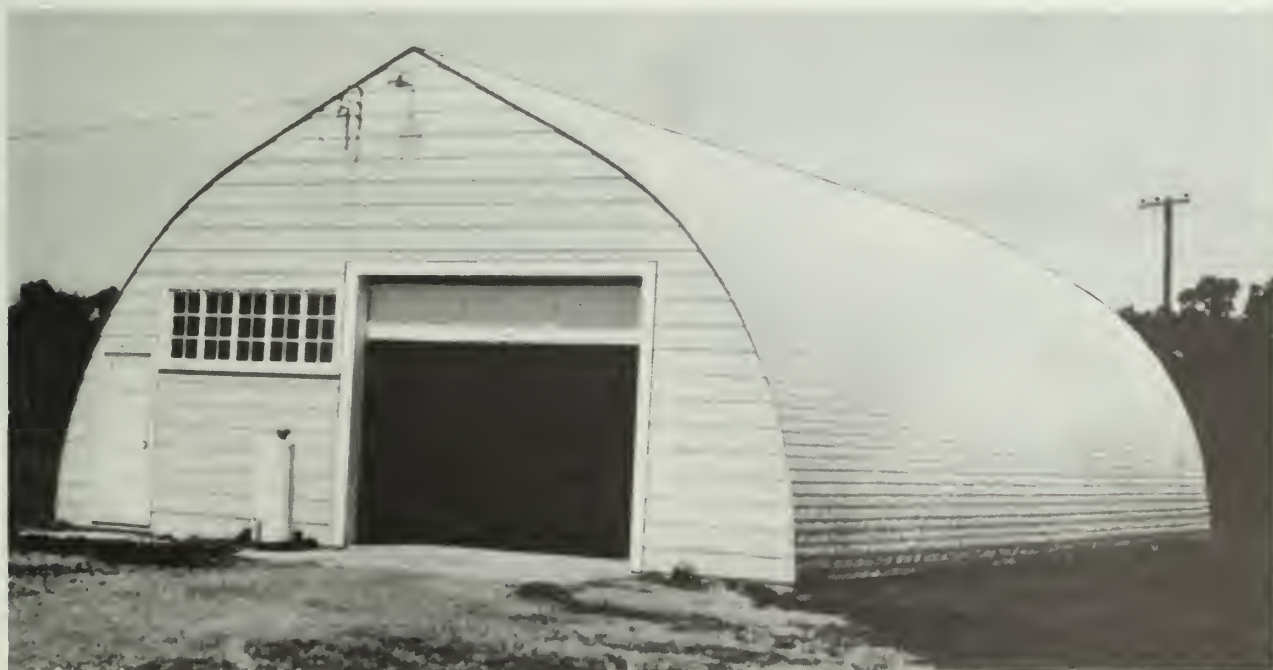
Figure 3 A standard arch rafter farm workshop
