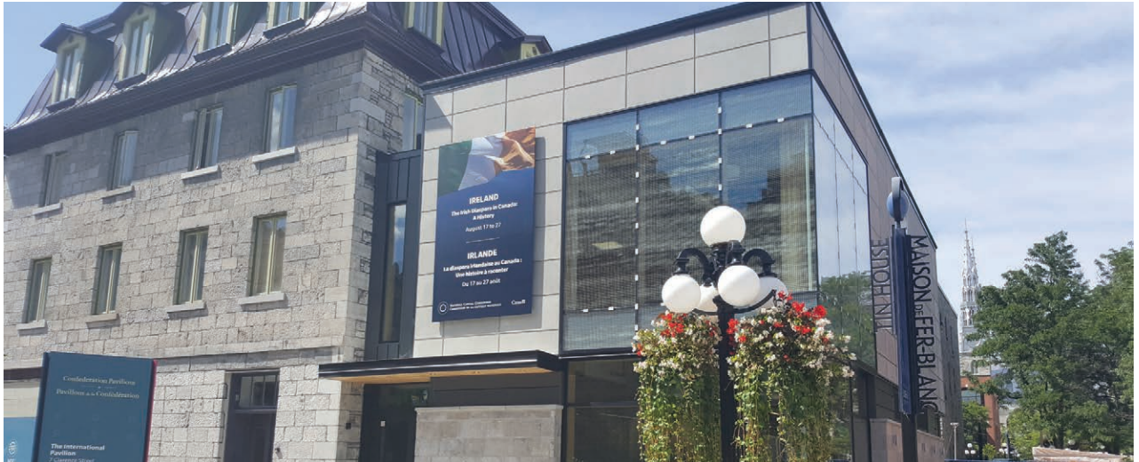
Bird-safe windows at the Confederation Pavilion at 7 Clarence Street.
