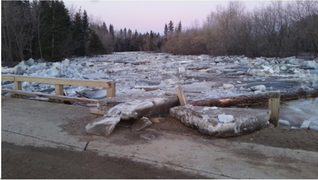
Figure 7 – Ice jam damage to bridge, Torch River, Manitoba 2017 (Regional Municipality of Torch River)
