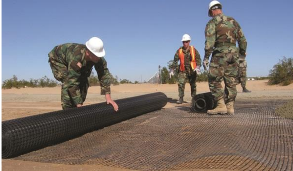
Figure 7: Deployment of a 'biaxial' geogrid 14 .
