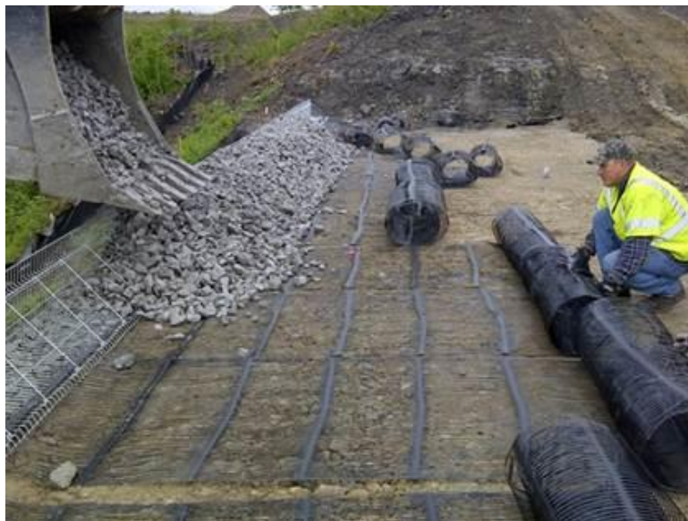
Figure 6: Deployment of a geogrid 13 - this one is of the ‘uniaxial’ type.
