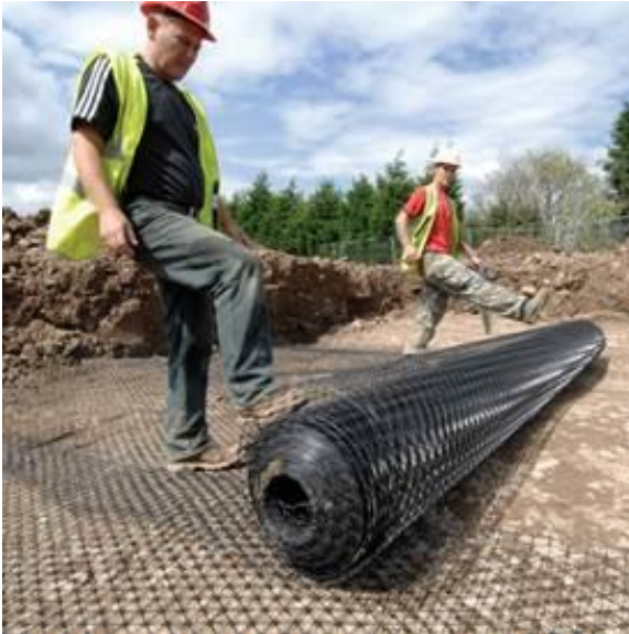
Figure 8: Left) Field deployment of a 'triaxial' geogrid 17 . Right) Schematics showing the load distribution exerted by a tire onto the supporting medium and the relevance of a triaxial material to compensate for strains in all directions.
