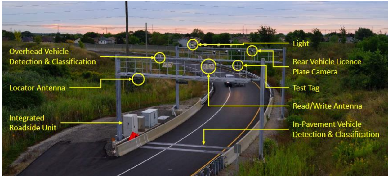
Figure 21: Typical infrastructure for AETC open road tolling (407 Express Toll Route in Canada [180]).
