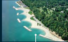
COASTAL & MARINE STRUCTURES
