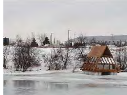
First prototype buoyant foundation built at University of Waterloo
