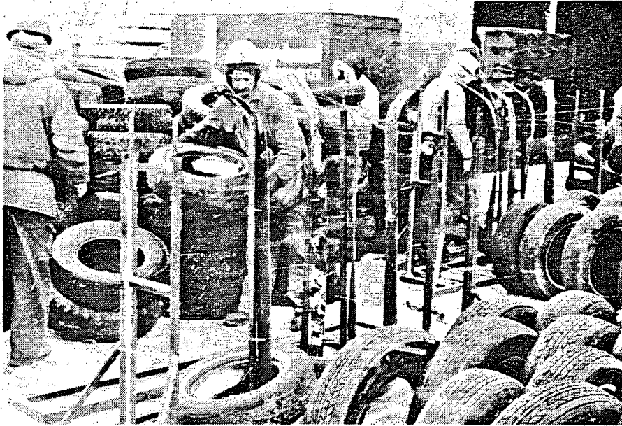
Figure 5. Tire frames used to assemble modules.
