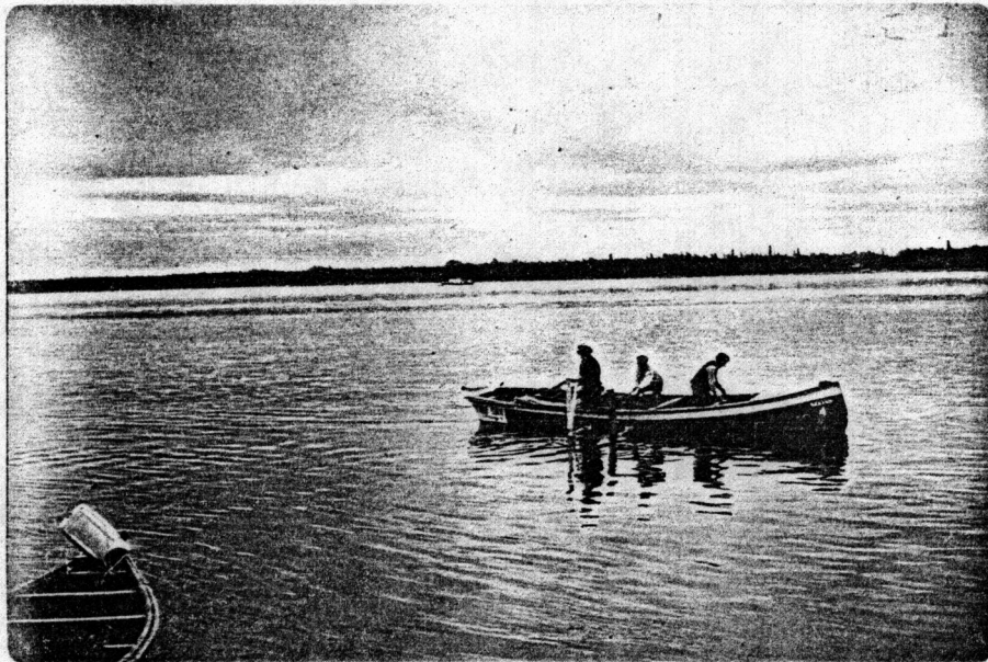
SUBMERSING ROCKFILLED CRIB
