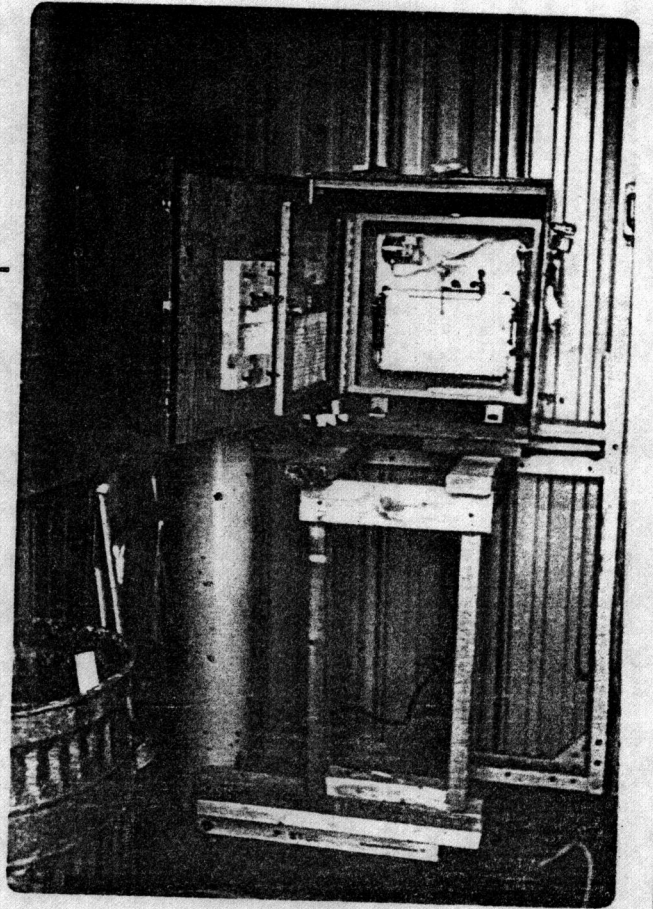
INSTALLED OTTBORO TIDE GAUGE
