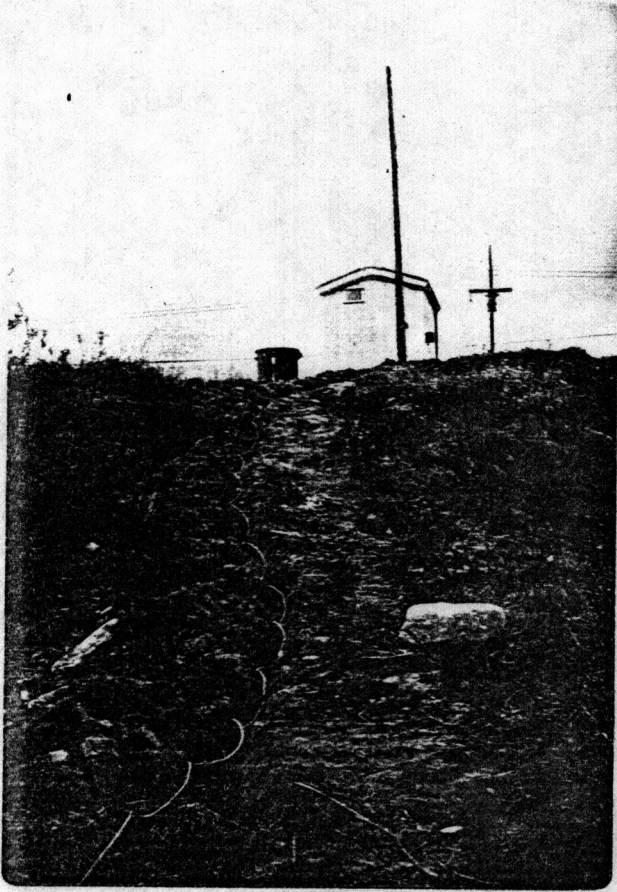
TRENCH FOR TUBING BELOW "GAUGEHOUSE"
