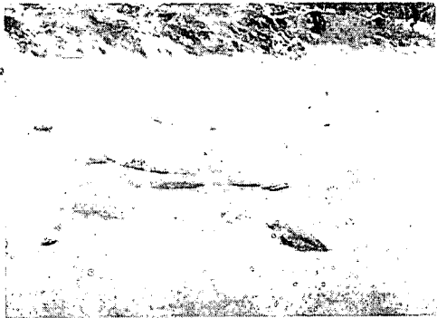
u/s side of Bothwell W. Bridge, looking toward Right Bank; 0900 h, Jan. 8, 1981. Note rough surface of ice cover.
