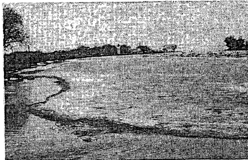
Toe of jam at 1400, Feb. 22, 1981. Looking d/s. Note relief of "rubble".
