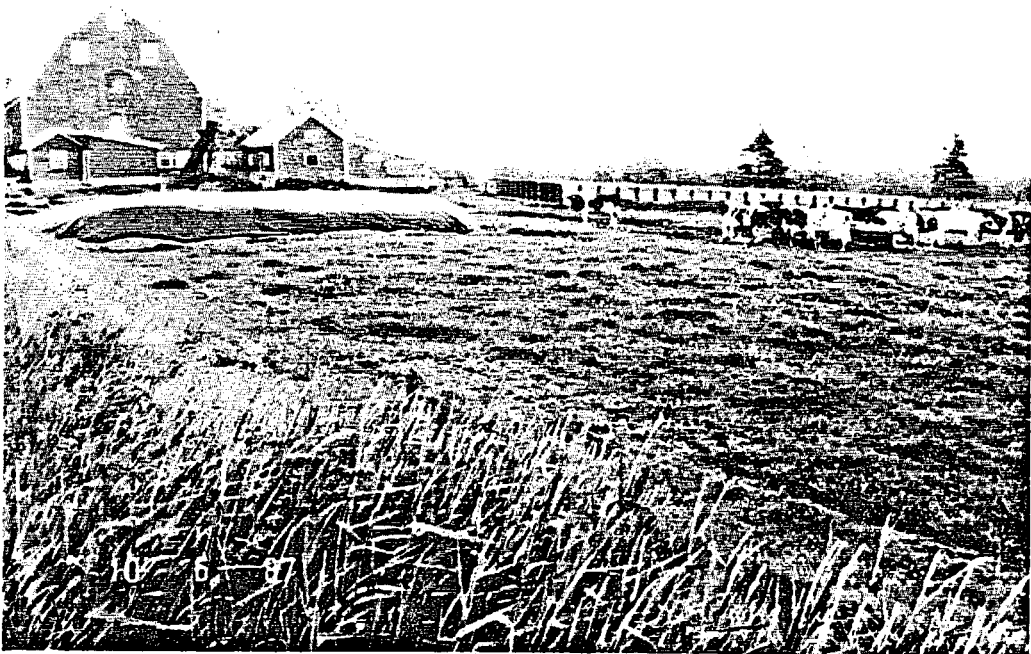
Plate 14. These covered piles limit materials reaching the water course. This photograph was taken near the community of Parker Road.
