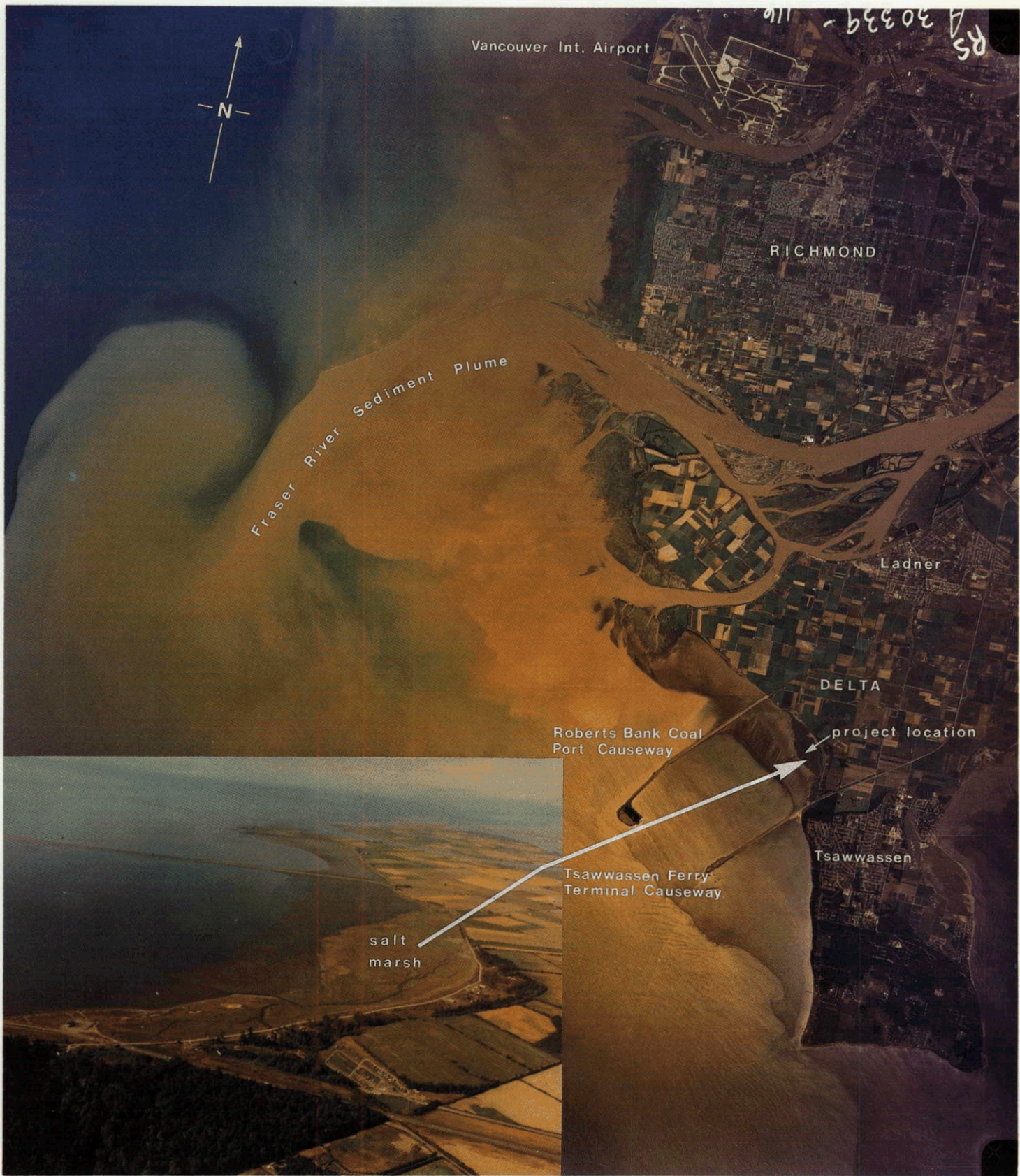
FIGURE 1 Location map of the Tsawwassen Indian Reserve Flood Control Works (aerial photo date 1971). Inset aerial photo (dated Sept. 27, 1974) looking north at the Tsawwassen salt marsh prior to 1975 dyke construction. The salt marsh is west of the Indian Reserve Road and bounded to the north and south by the Roberts Bank and Ferry Terminal Causeways. Photo courtesy of Delta Municipality
