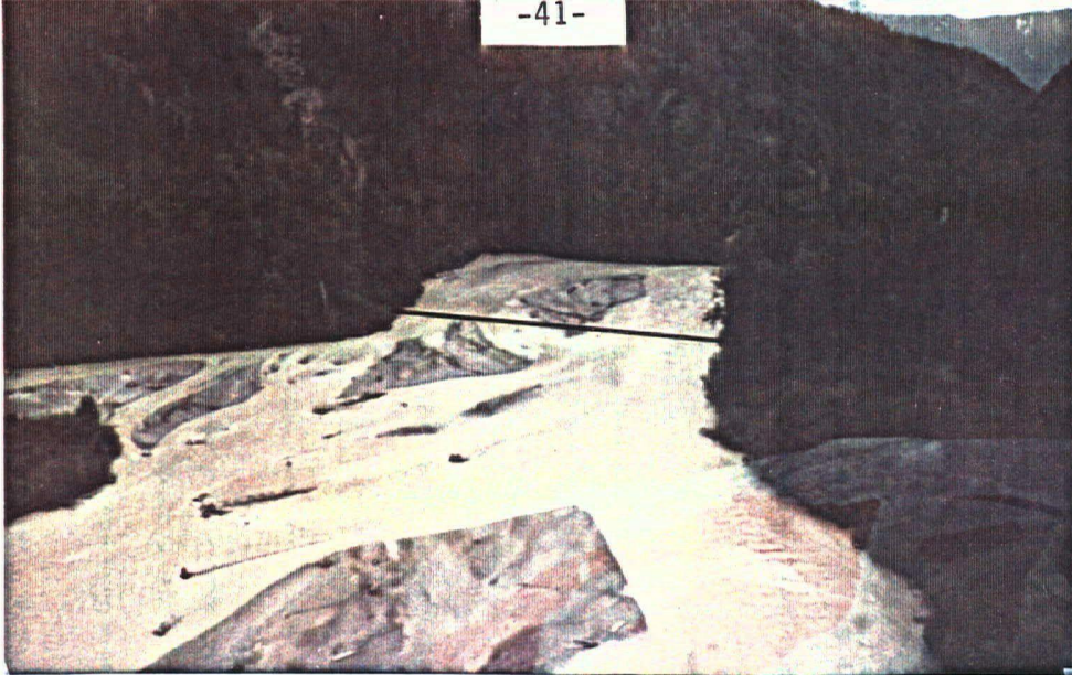
Cableway 200 Metres Upstream from Recorder Location
