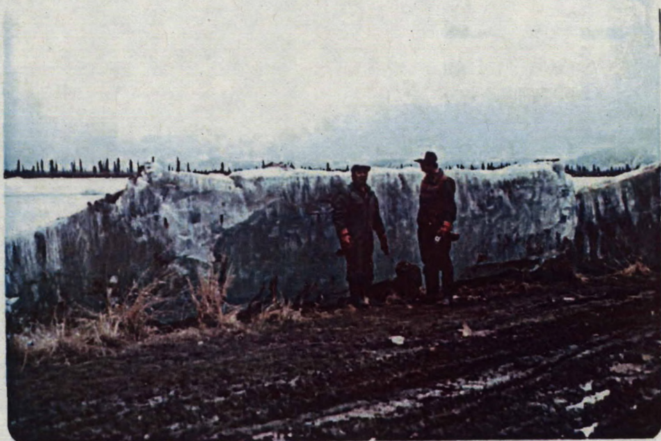
Photograph 14. Ice shove on road in front of old HBCo. store, Aklavik, 02 June 1982, 1350 MDT (black ice thicknesses between 1.5-1.8 m).
