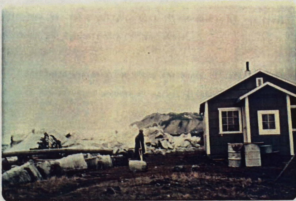
Photograph 9. 1964 ice shove on lower terrace of Fort Norman Settlement, 28 May 1964.
