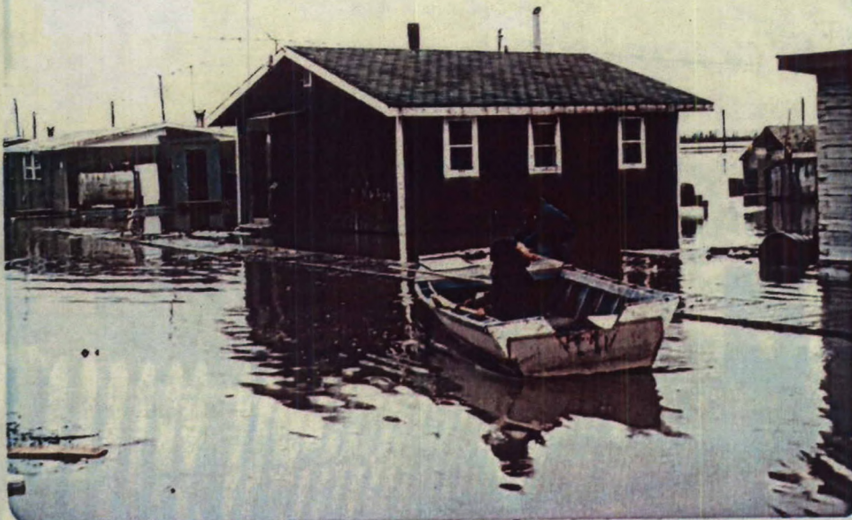
Photograph 15. Floodwaters inundating main road in Aklavik, viewed 1 block north of HBCo. store, 02 June 1982, 1305 MDT.
