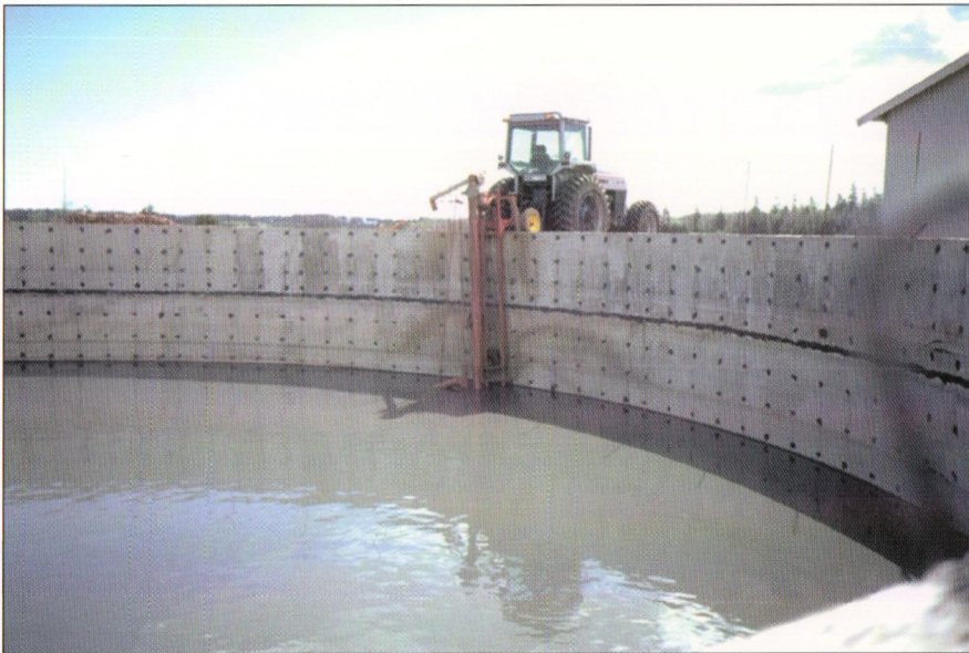
Liquid manure storage - circular concrete tank.
