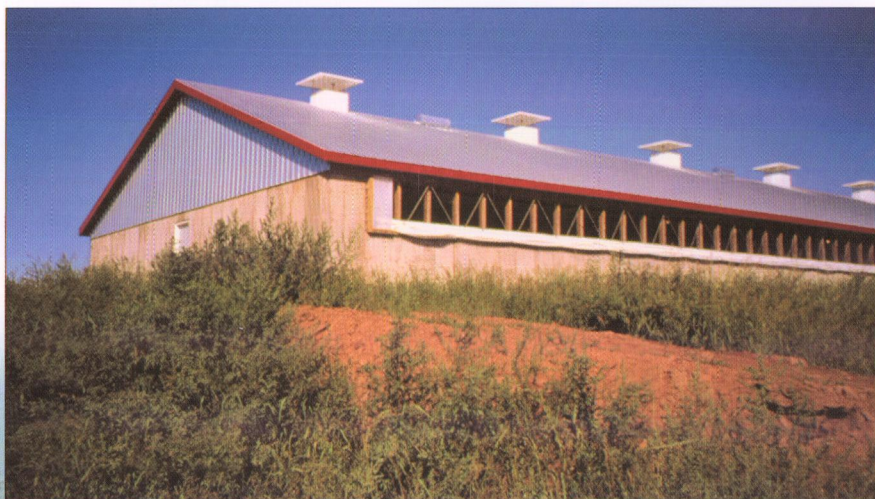
Roof exhaust outlets to maximize air dilution.
