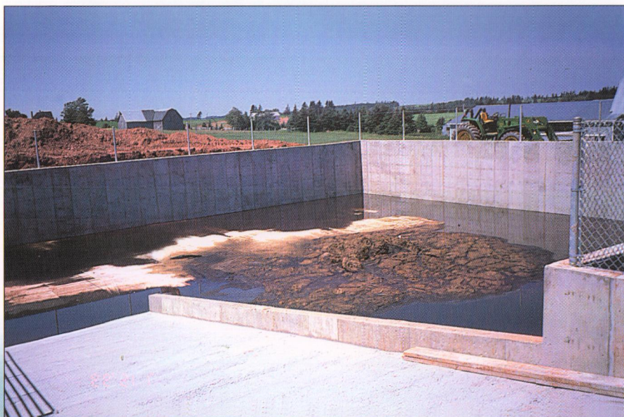
Curbed concrete manure storage with safety fence.
