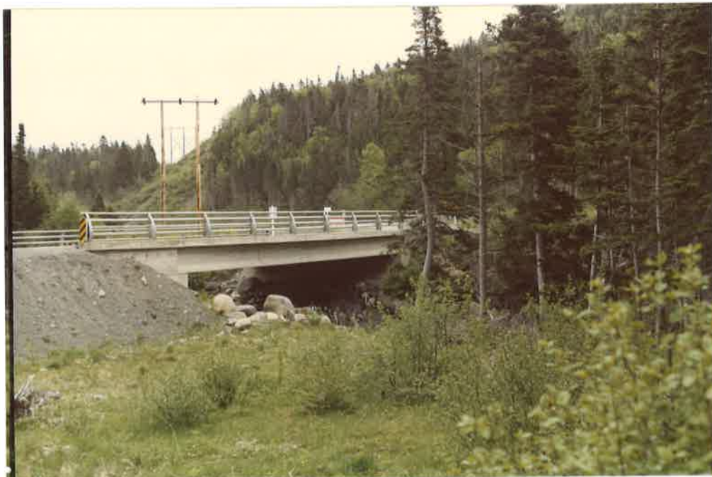
BRIDGE IN GLENBURNIE AREA
