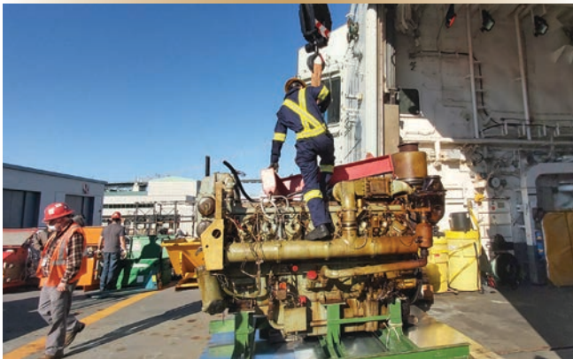
Figure 2a and b. A legacy MWM 602 engine is rigged and ready to be lifted out of the AAMR, and then craned ashore.
