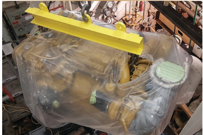
Figure 4. A new Caterpillar CAT ACERT32 engine, still in its protective wrap, is rigged into the AAMR. Note the tight clearances.
