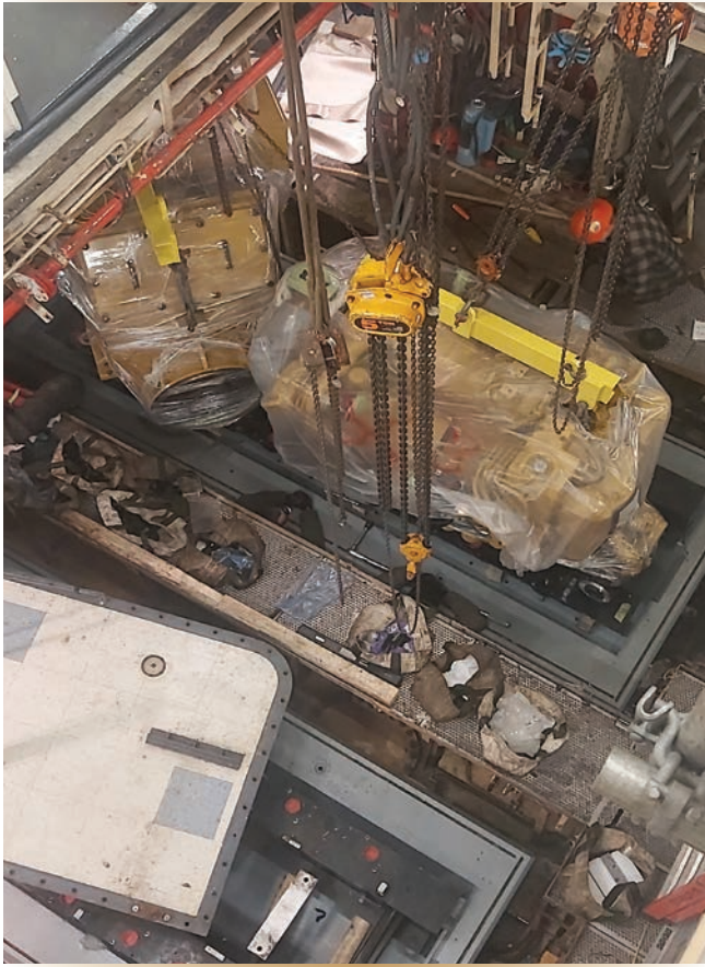
Figure 5. A new engine and generator are positioned on the machinery raft.
