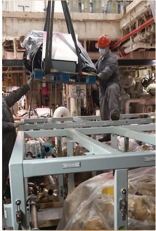
Figure 6. In the foreground, the new engine enclosures can be seen mid-assembly.
