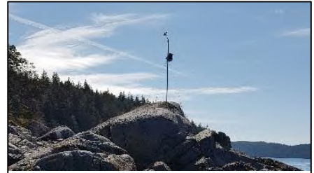
Figure 1. Weather station installed at remote site.
